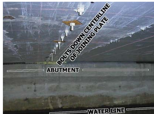
Figure 4. View of Underside of Composite Bridge Deck, Looking North with Centerline Joint
