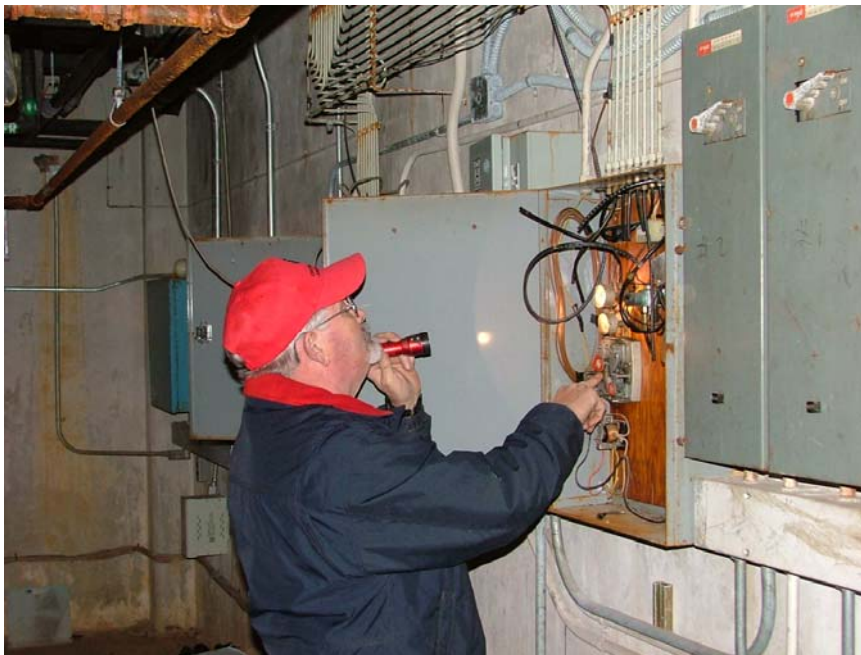
Figure 1. Antiquated pneumatic style controls are abundant at Fort Bragg.
