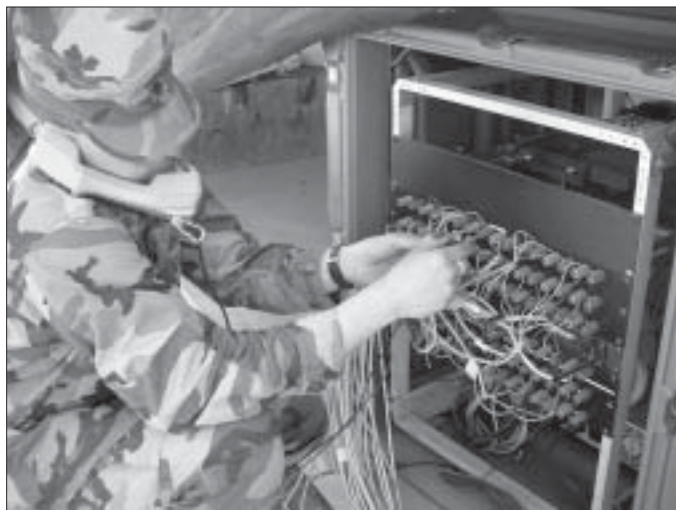
Figure 18. SPC Dennis Braun tests extension lines on the Warrior PBX during Exercise Native Atlas '02.
