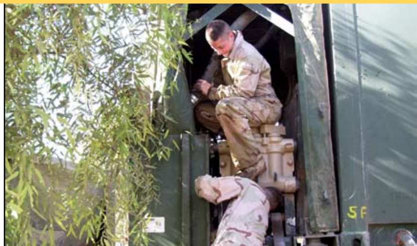
Two Soldiers of the maintenance section fix a high-pressure pump on one of the 3,000-gallons-per-hour ROWPUs.
