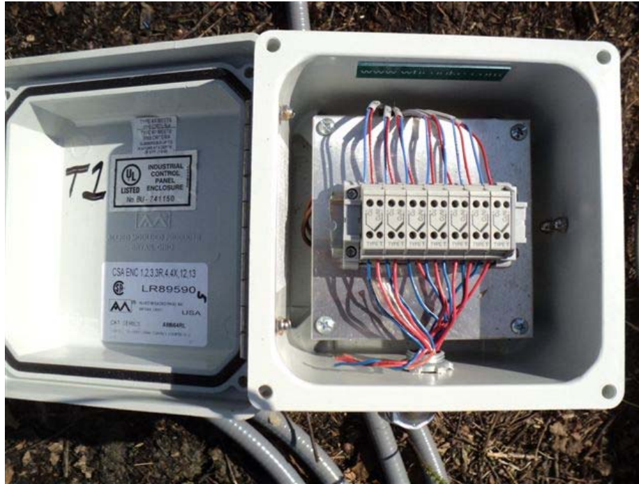
a. Thermocouple (TCP4) box showing close-up of wiring.
