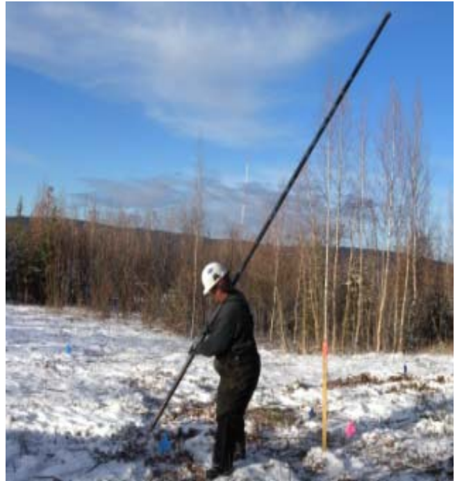
b. Heater casing being placed into hole.
