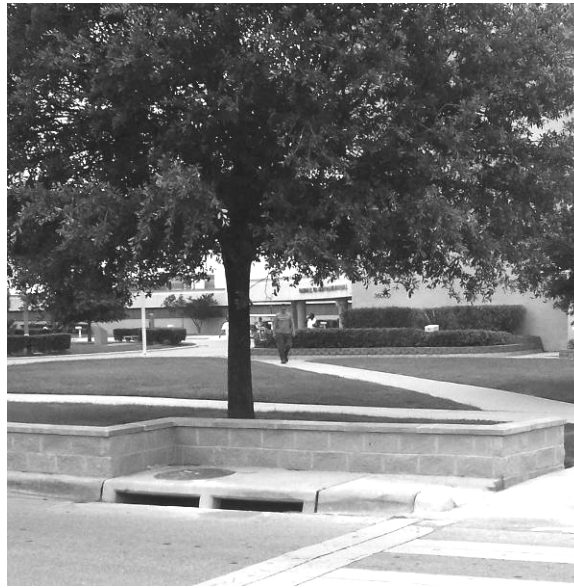
Figure 4. Place barrier walls at the curb where there is already a change in site elevation (DA 2005).
