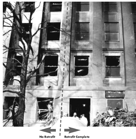
Figure 39. Pentagon immediately after September 11, 2001, showing intact blast-resistant windows at right.
