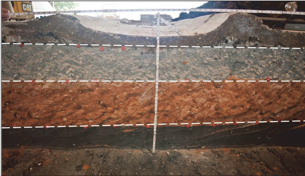
Figure 67. Foamed Asphalt South Trench (STA 0+16).
