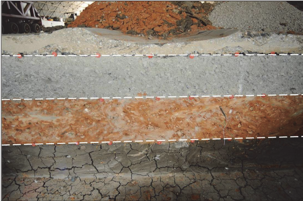
Figure 71. Evotherm™ 3G South Trench (STA 0+16).
