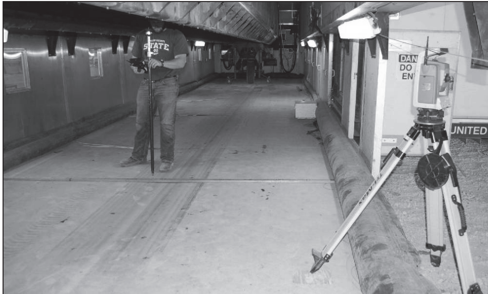
Figure 15. Cross-section readings with robotic total station.
