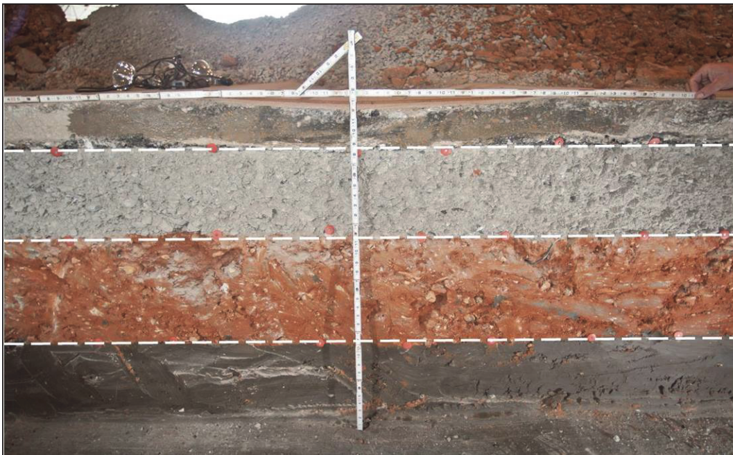
Figure 66. HMA North Trench (STA 0+36).
