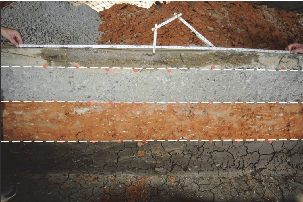
Figure 70. Sasobit® North Trench (STA 0+36).
