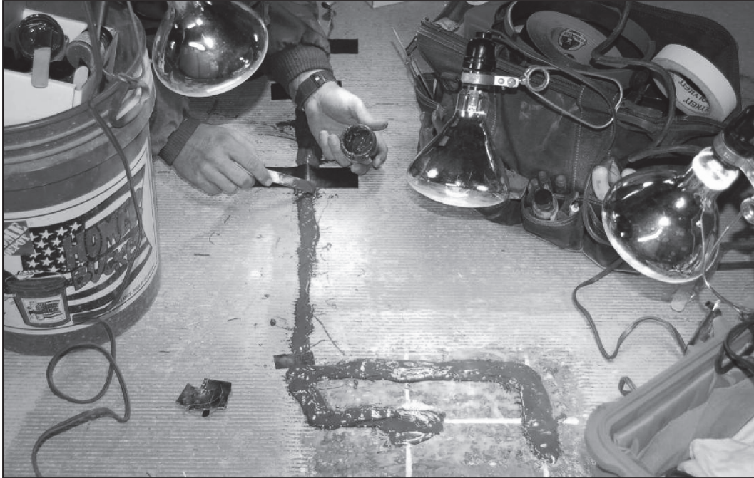
Figure 8. Applying protective coating to SSGs and lead wires.
