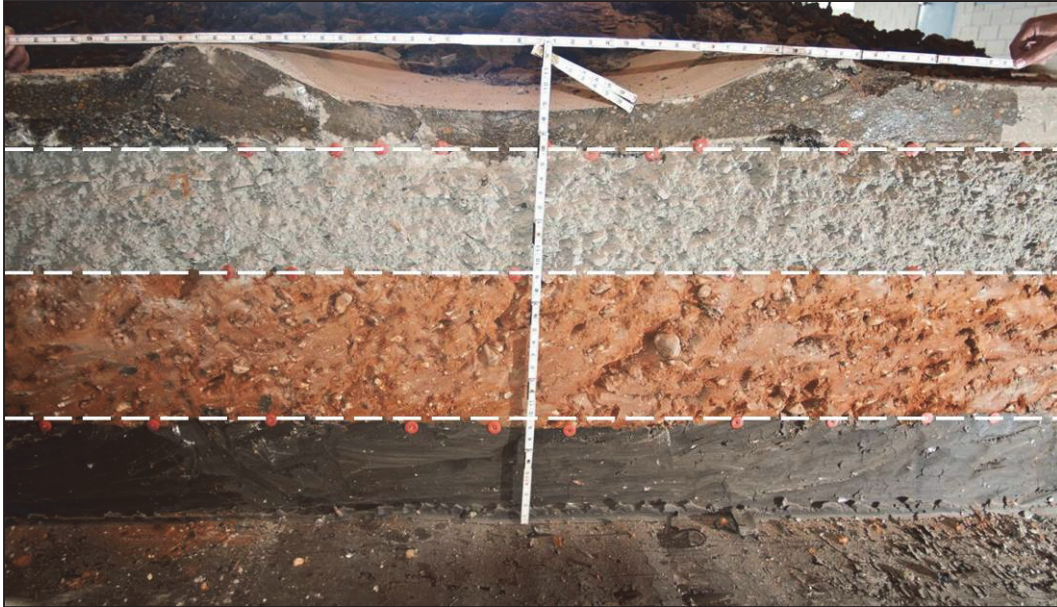
Figure 65. HMA South Trench (STA 0+16).
