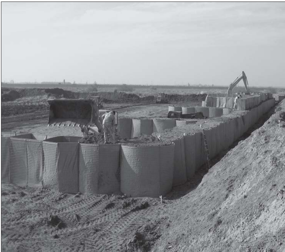
HESCO Bastion Concertainer® units surround an ammunition holding area.
