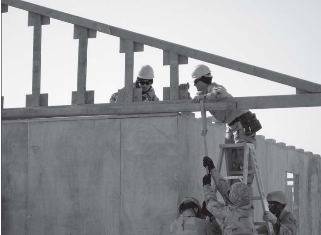
Soldiers and Airmen build a tactical operations center for the 1st Cavalry Division.
