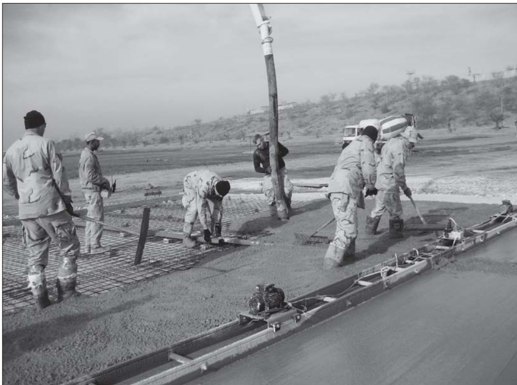
Engineers place cement pads in preparation for surge forces.
