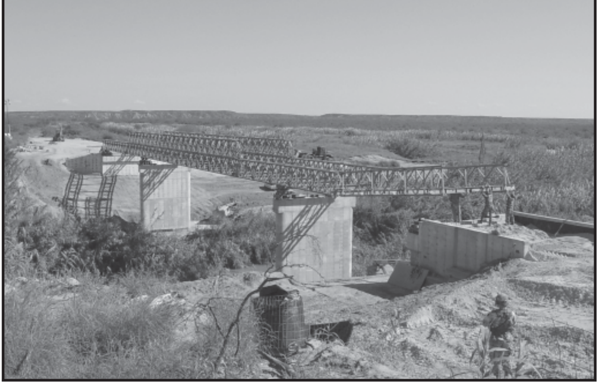
Finished bridge launch
