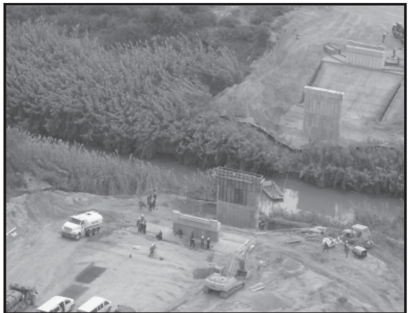
Aerial view of scour apron preparation
