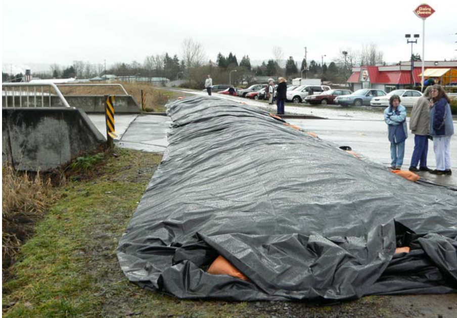
Photo 6.6. Coweeman: quarry waste wrapped in plastic sheeting across Grade Street
