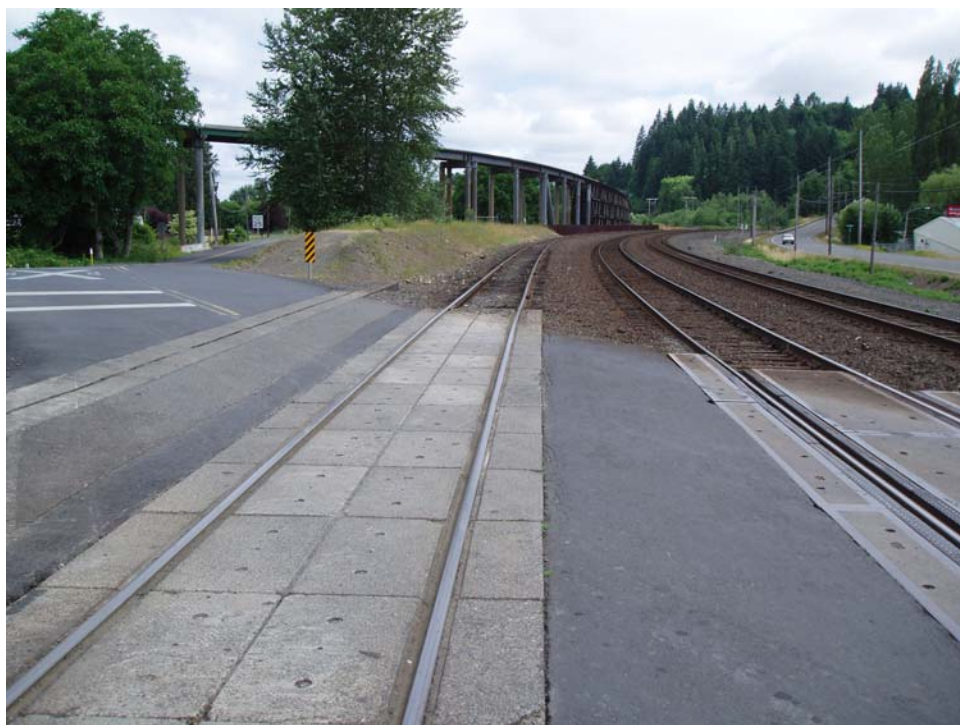
Photo 5.1 c. Kelso reach KL1, road crossing
