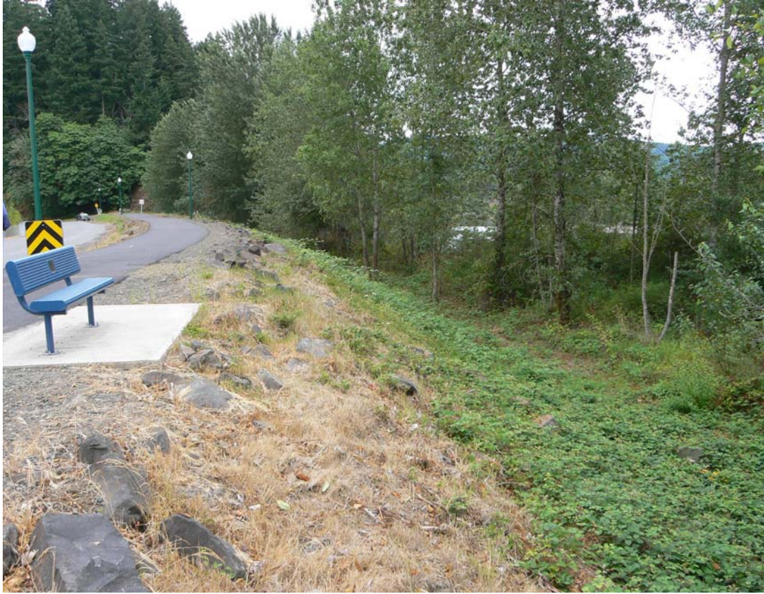
Photo 2.8 b. Castle Rock reach CR8, riverward slope with riprap to levee crest
