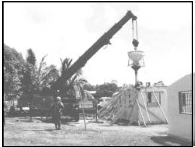
Using a concrete bucket to fill the panels
