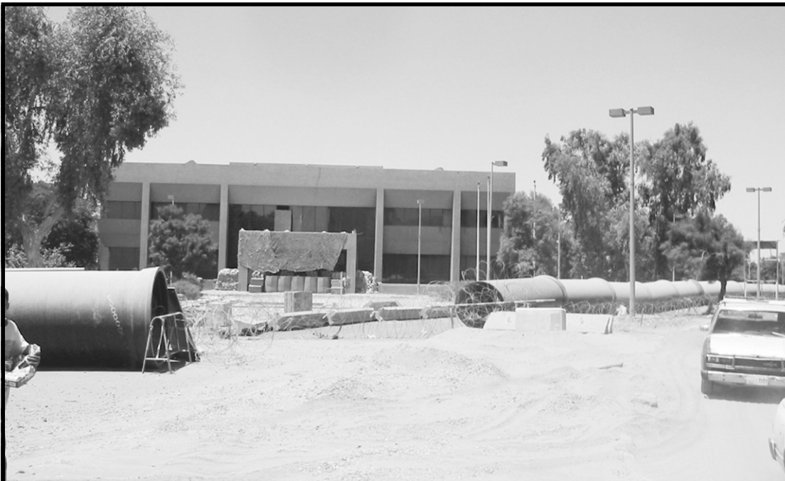
Storm water piping was used as a barrier for the perimeter of the compound.
