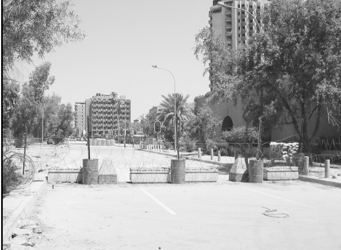
A barrier in front of the Palestine Hotel in Baghdad was constructed using 55-gallon drums with pickets and concertina wire.
