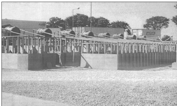
Figure 8. Shower Area Where Hospital Corpsman Cedergren Was Electrocuted (From Navy Photographs)
