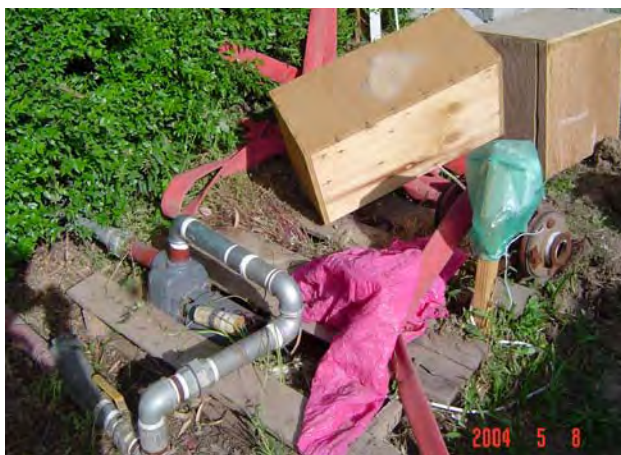
Figure 5. Covers for Pump and Fuse Box in Area Where Specialist Whitham was Electrocuted (From Navy Photographs)
