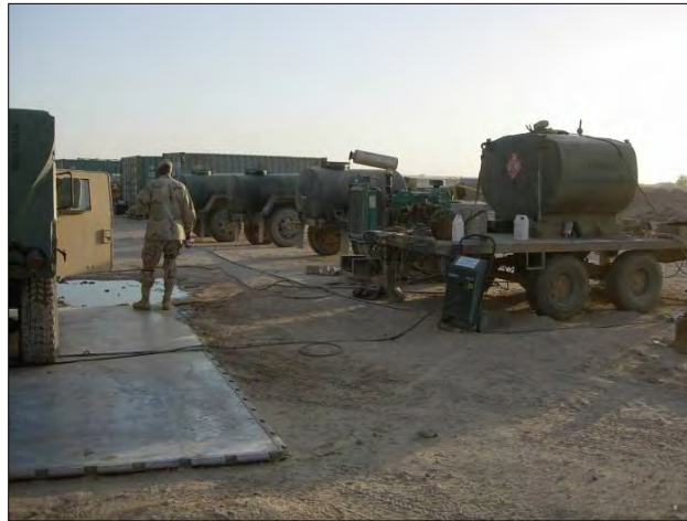
Figure 10. Area Where Sergeant Everett Was Electrocuted (From Army Photographs)
