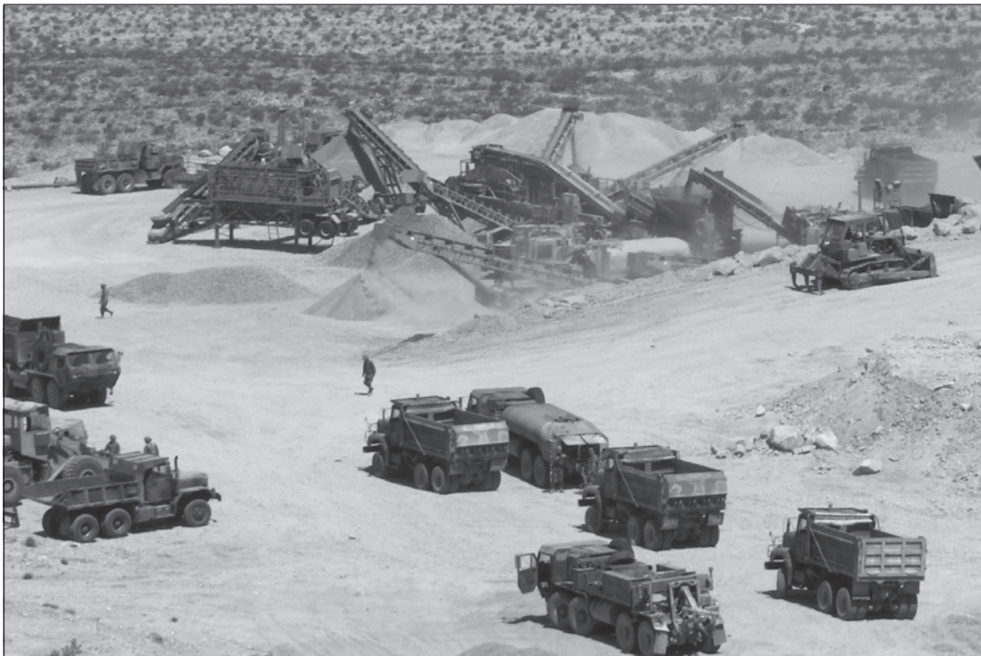
Quarry site where gravel is produced for NTC construction projects
