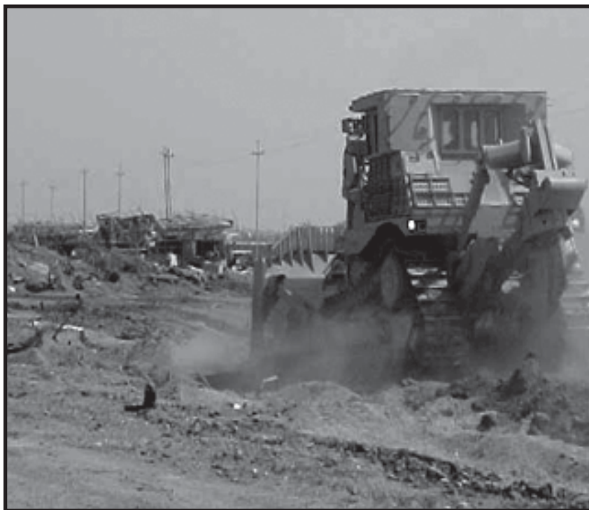
The mighty D9 dozer clears rubble in preparation for a reconstruction mission.
