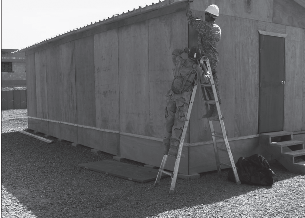
A Seabee and a Soldier work side by side hanging trim on a SWA hut.
