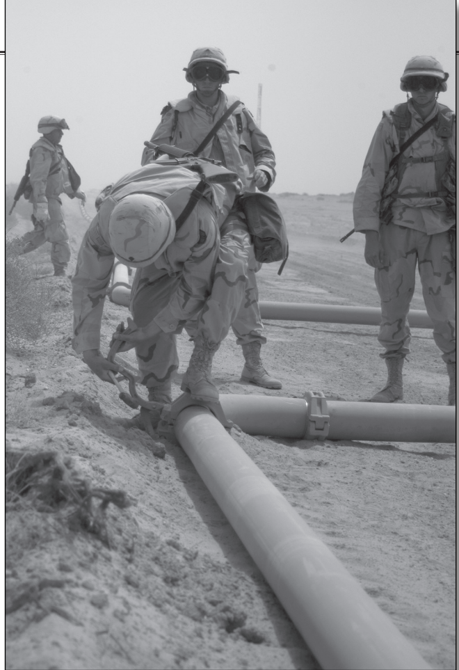
Pipeline engineers attach redesigned couplings that made laying pipelines much easier.
