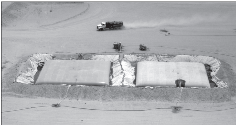
The system using inflatable blister bags was developed in the 1950s and was still in use during the 2003 invasion of Iraq.
