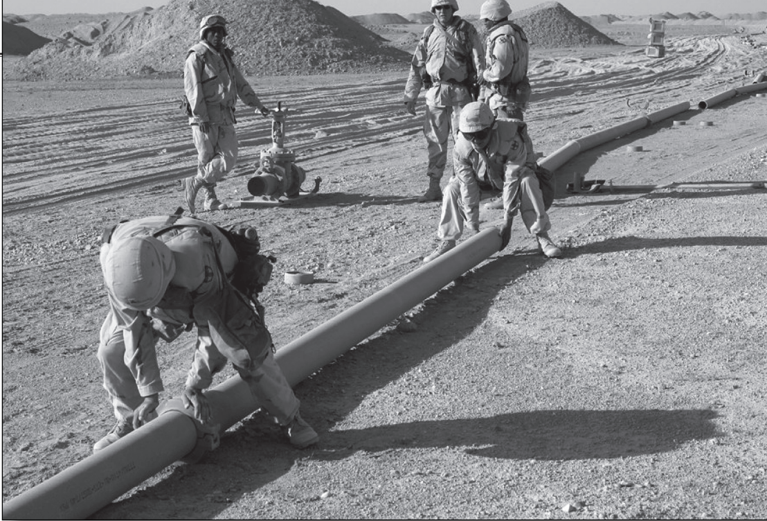
A crew positions the pipe before installing a gate valve.
