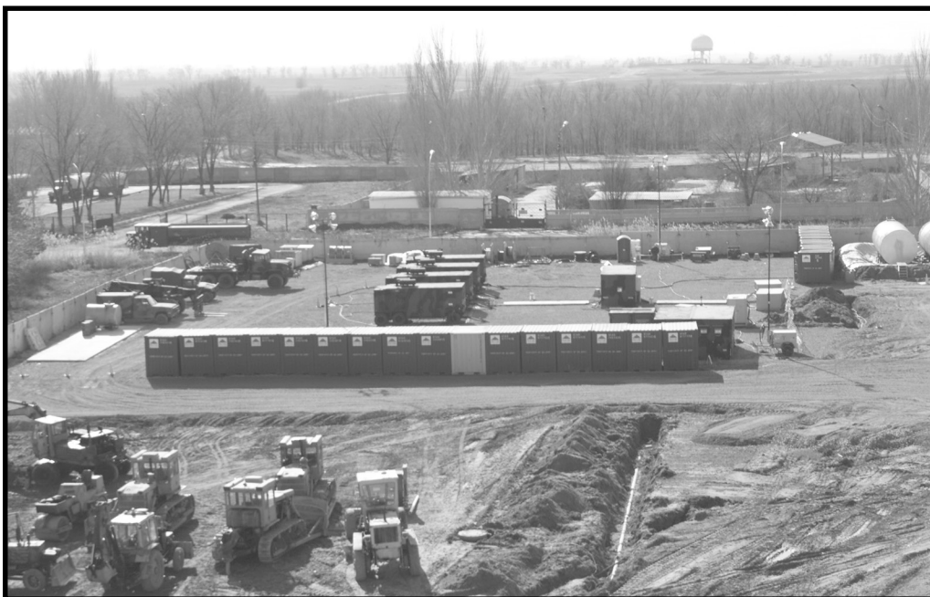
Power plant installed in Kyrgyzstan
