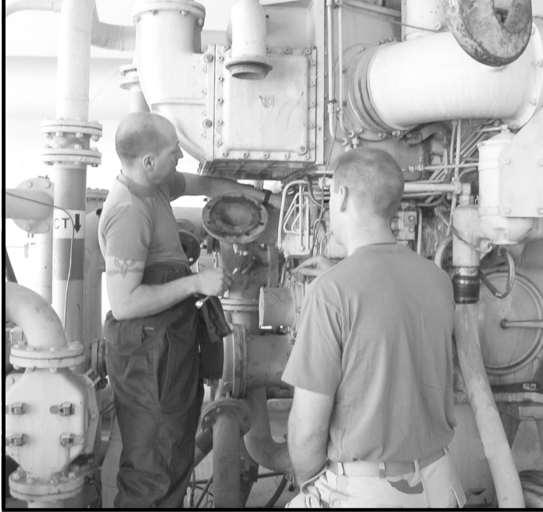
Two prime-power soldiers repair an Iraqi generator.
