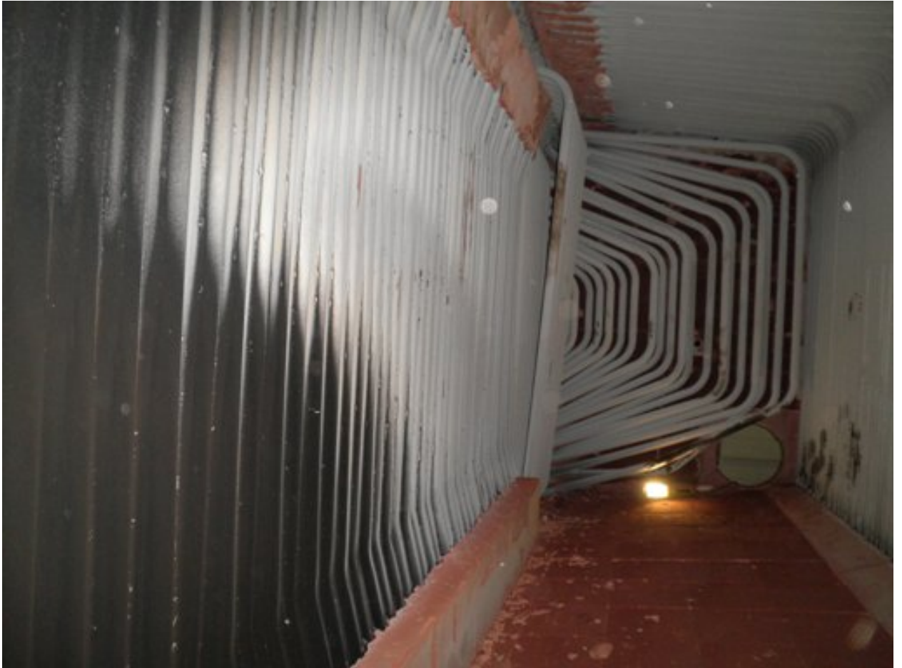
Left Side Wall Water Tubes toward Rear of Furnace
