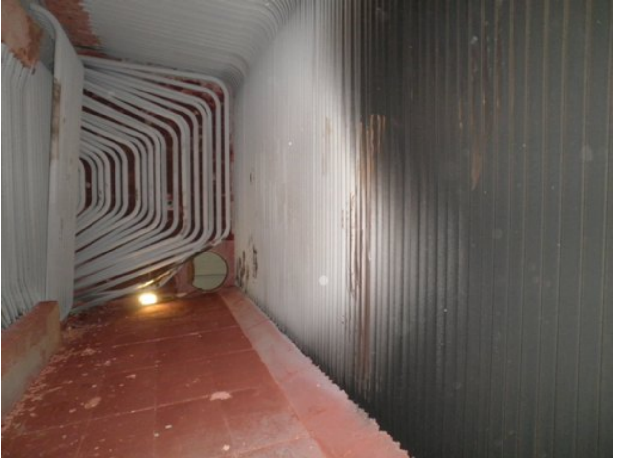
Right Side Wall Water Tubes toward Rear of Furnace
