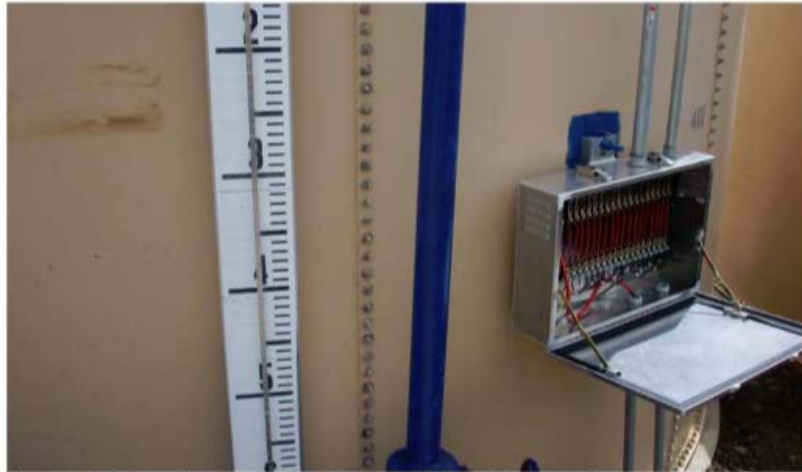
Figure 6: ICCP anode system junction box (opened). Note also external tank water level gauge.
