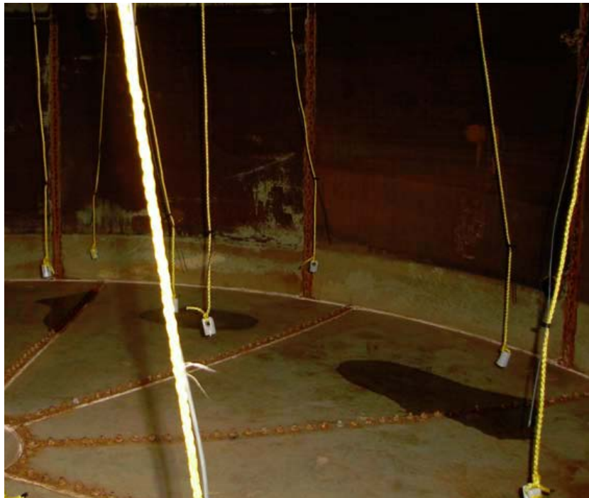
Figure 10. Anodes suspended and stabilized with ceramic insulators and nylon rope.
