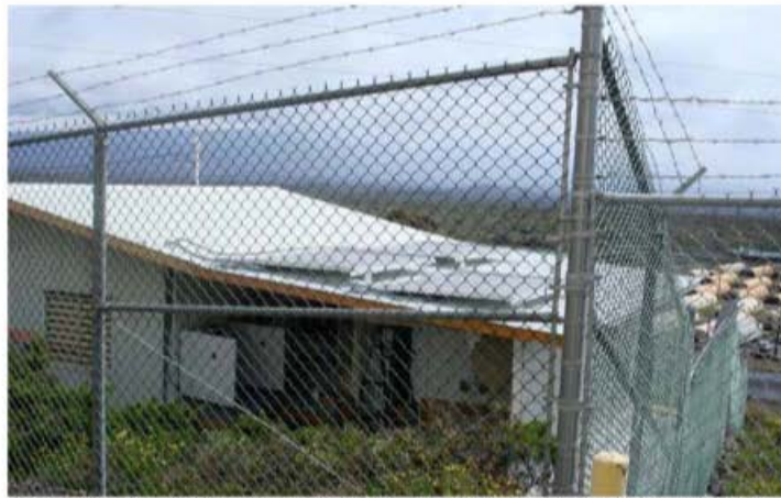
Figure 18: Solar Panels on top of building. Each panel consists of three 130 Watt PV modules connected in parallel with each other. There are three panels.
