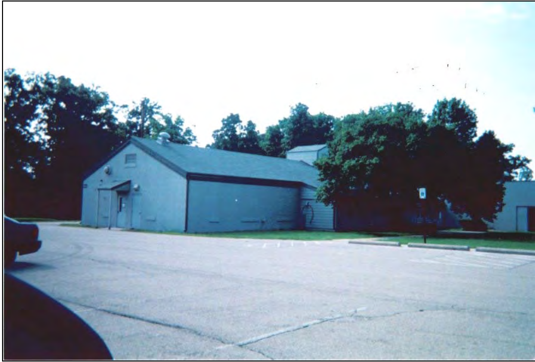
Photograph #9: Building 20682, proposed for demolition.
