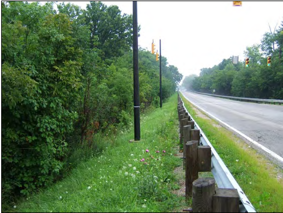
Photograph #13: Location where the proposed gate and turn lanes may be constructed on National Road.
