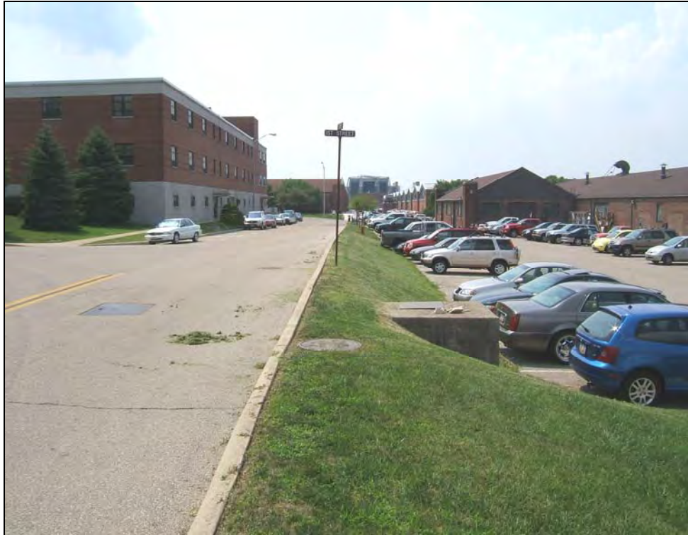
Photograph #23: Typical view of area of proposed wastewater line improvement in the Downtown District, along F Street.
