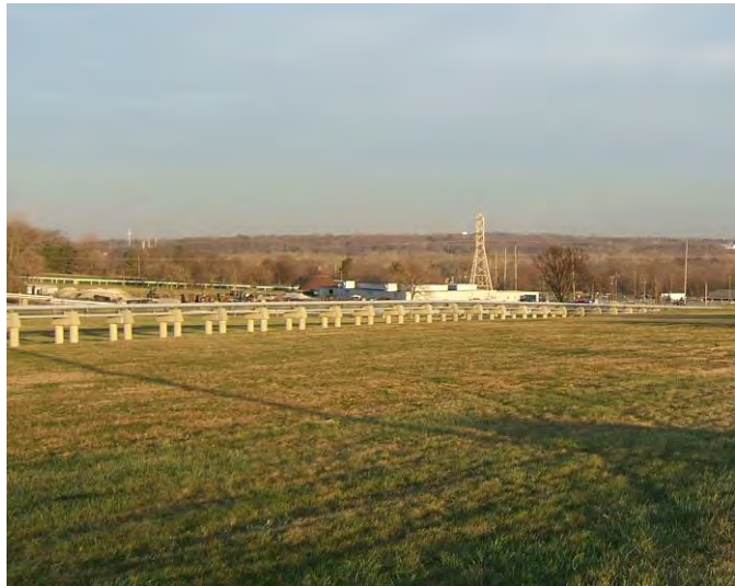
Aerial steam line “A” across the proposed HPW complex site.
