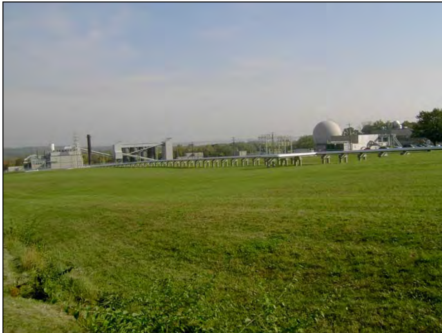
Photograph #6: Above ground steam lines in the proposed location of the AFRL/HPW Complex North (view to the northeast).
