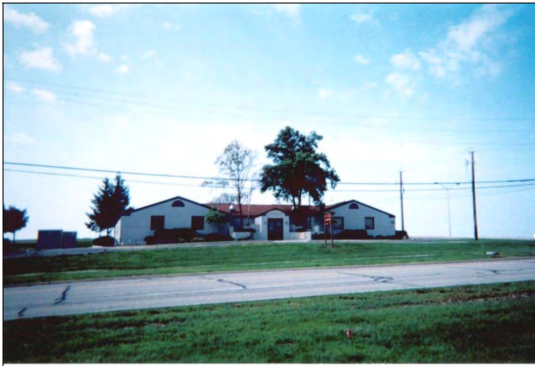
Photograph #8: Building 20430, proposed for demolition.
