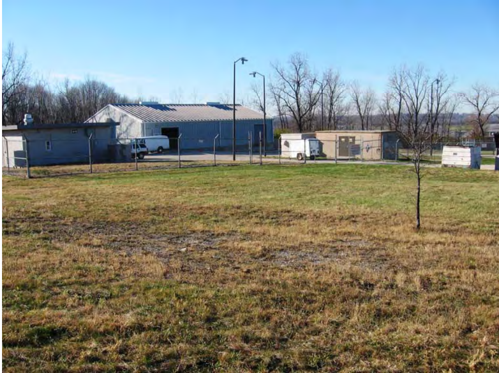
Photo 1: Looking south across site towards existing RCRA waste storage facility
