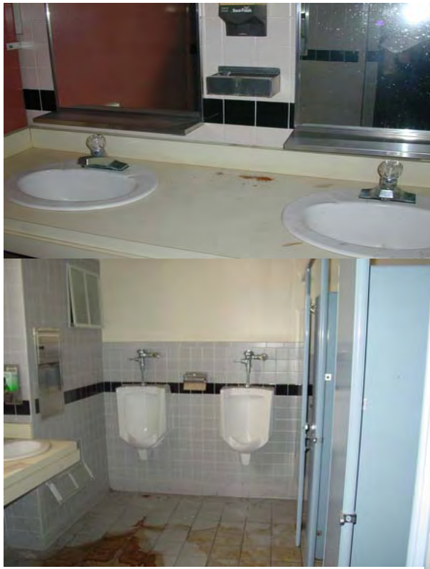
Photo 6: Typical Restroom to be Replaced
