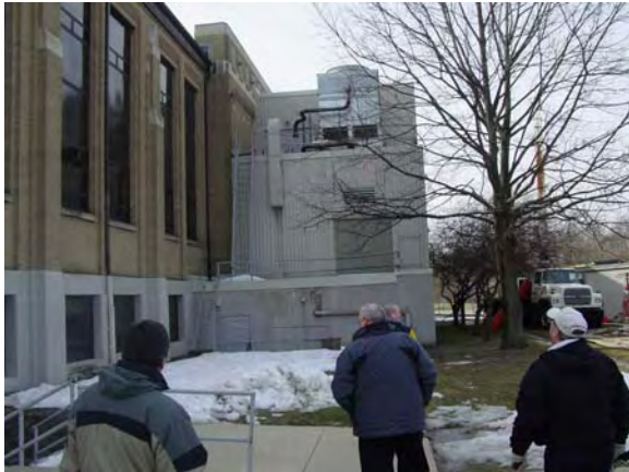
Photo 3: Mechanical Addition – North Façade
