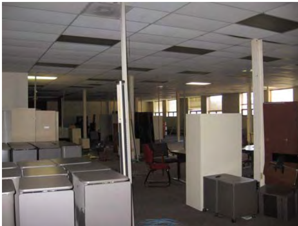
Photo 23: Existing Office Level 1
