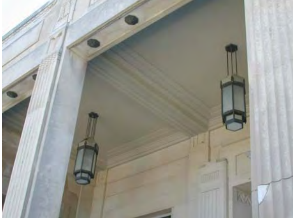
Photo 13: Entry Portico Ceiling and Lights
