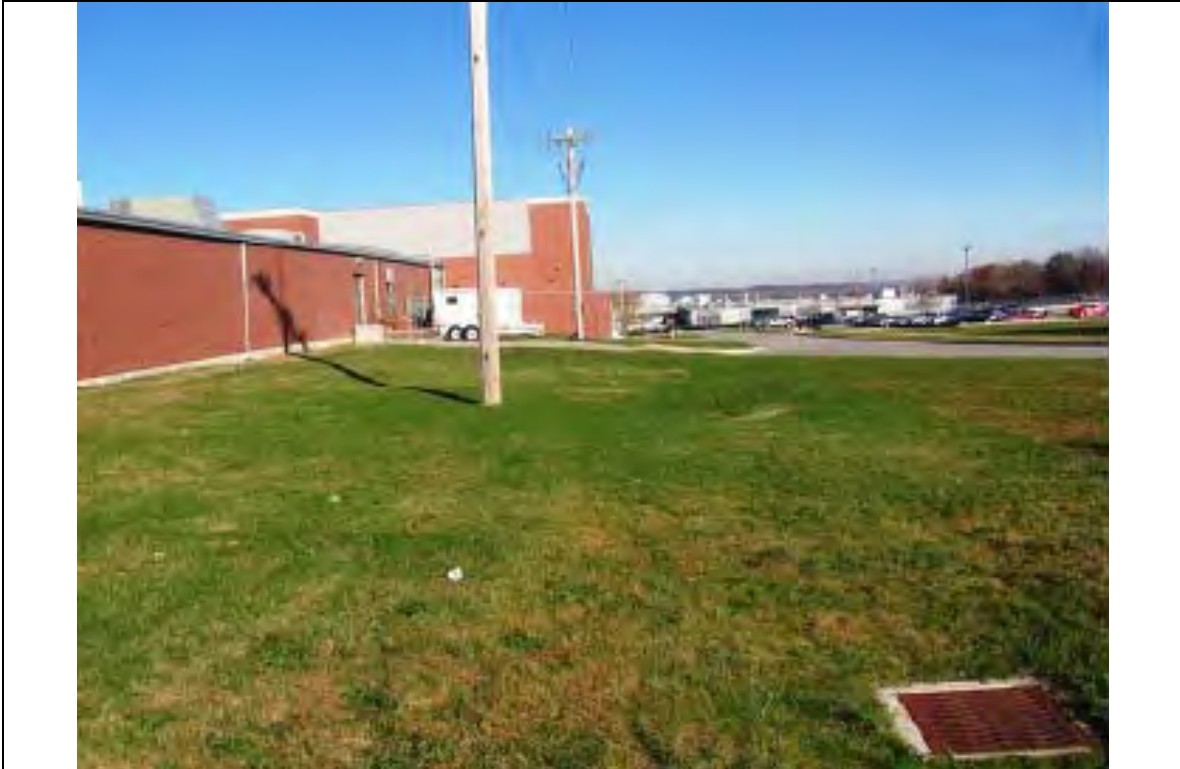
14. View north at site of proposed addition to Facility 20838.
