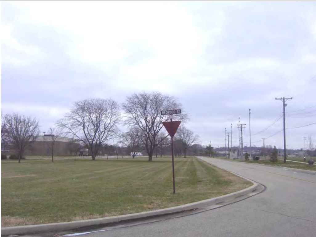
23. View of Redwood Street along north side of Pipeline Dormitory site.
