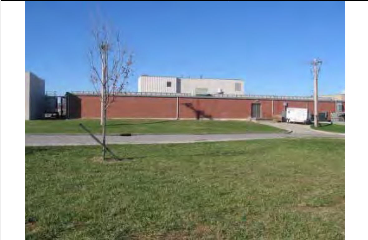
13. View west at site of proposed addition to Facility 20838.
