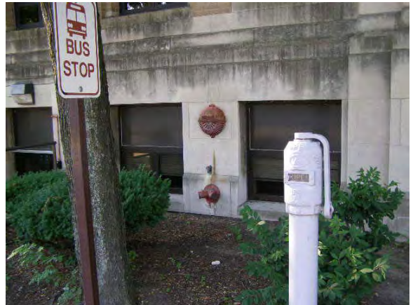
Photo 10: South Façade Limestone
