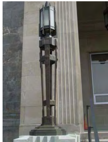
Photo 12: Exterior Entry Light Fixture
