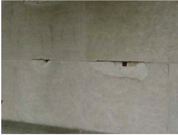
Photo 7: Limestone Repair
