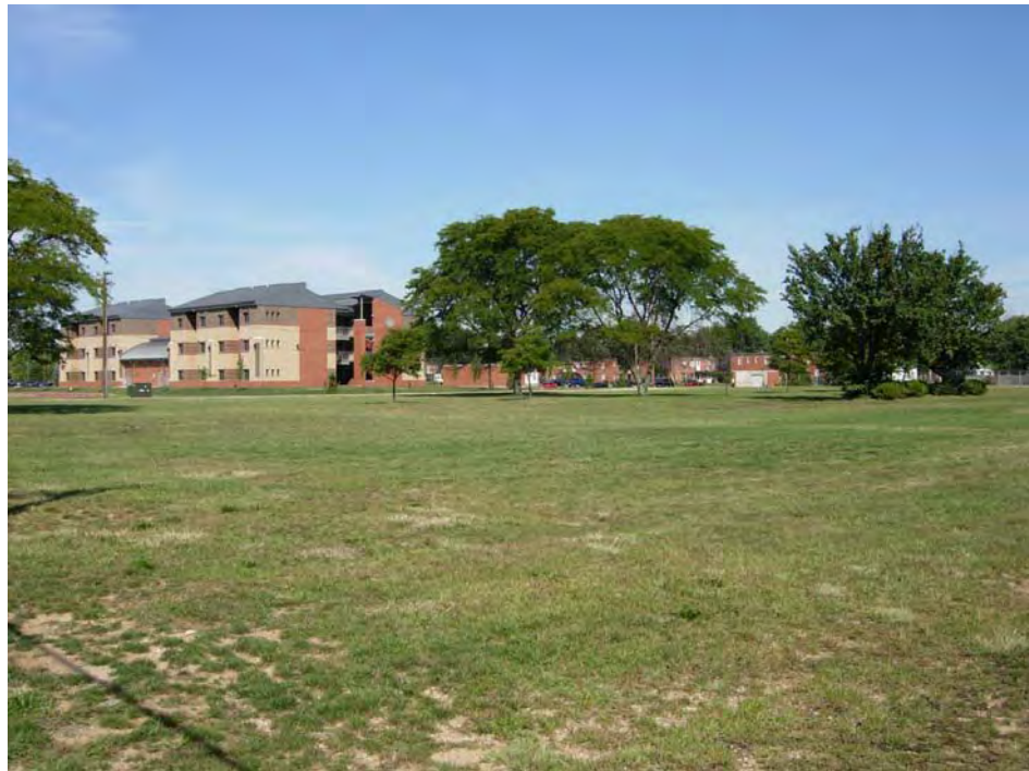
Photo 2: Looking north across site towards Dorm 31218
