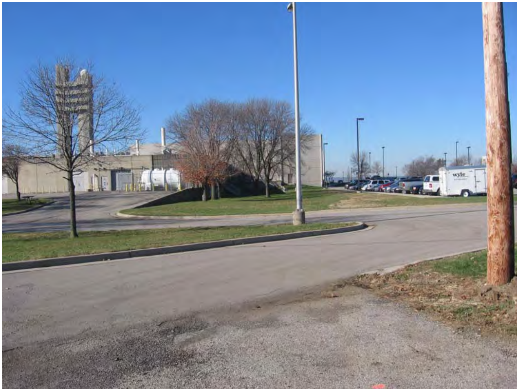
Photo 2: Looking west at east elevation of 20620
