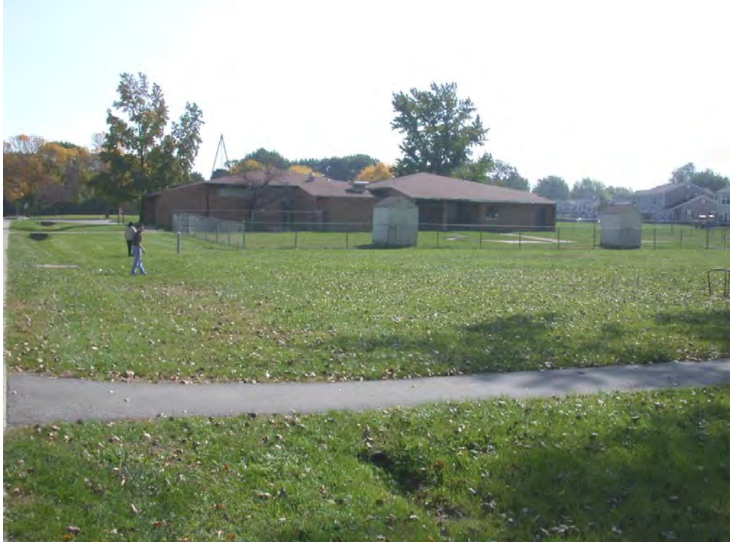
25. View of the proposed Chapel Life Center Addition site, from the northwest.
