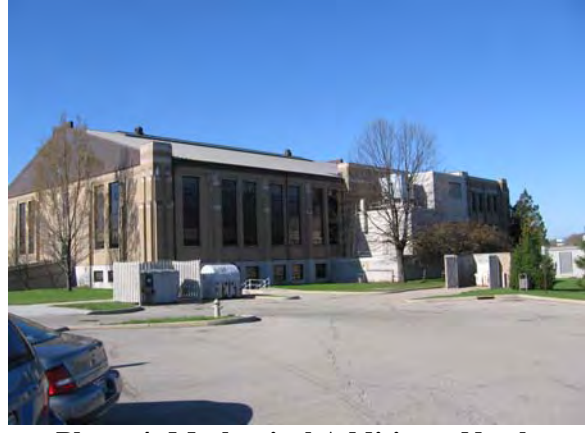
Photo 4: Mechanical Addition – North Façade
