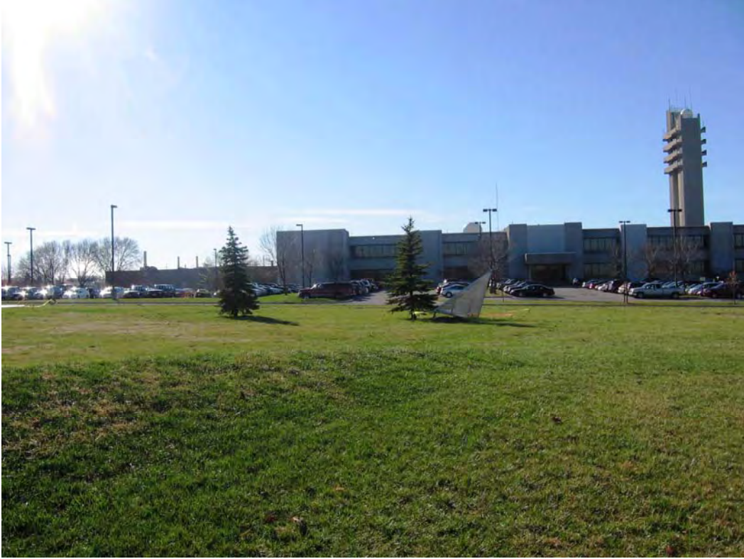
Photo 1: Looking south at north elevation of 20620
