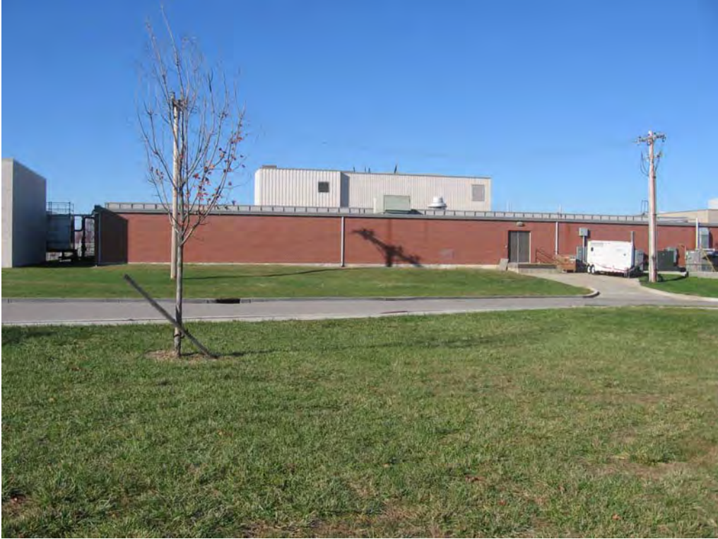
Photo 1: Proposed site looking west at southeast elevation of 20838
