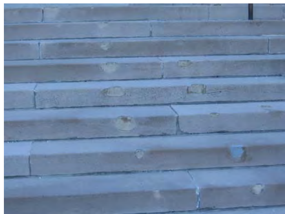
Photo 6: West Entrance Stairs
