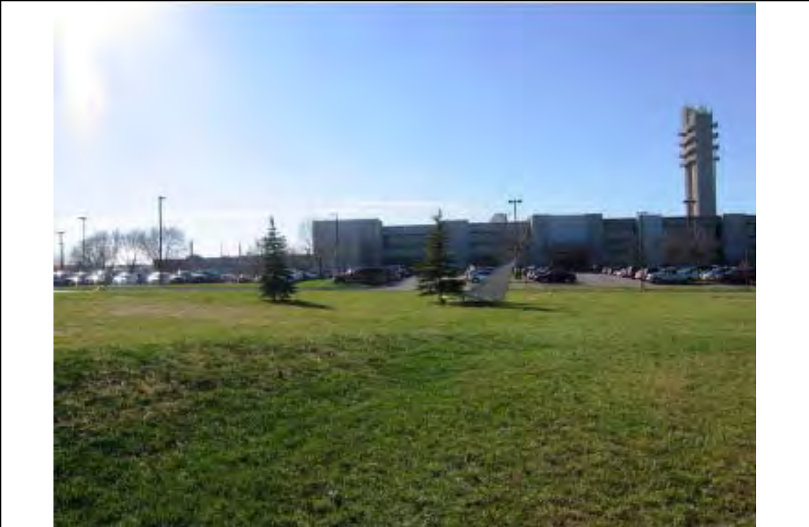
10. North side of Facility 20620
