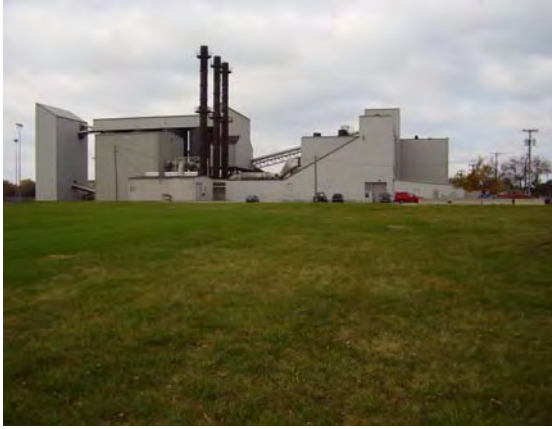
Photograph 1: View of the central and west portion of the Alternative 2 location and adjoining property (heating plant in the background), facing west.
