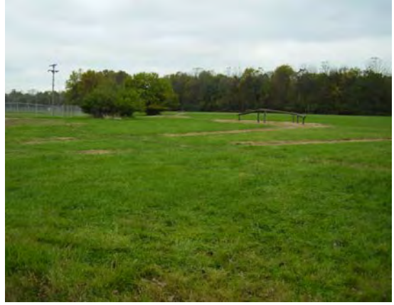
Photograph 8: View of the south portion of the Alternative 1 location and adjoining property (background), facing southwest.
