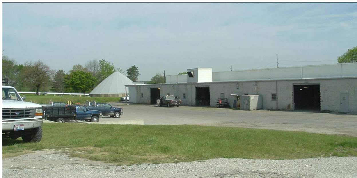
Figure 4-5: Southwest Façade of Facility 20745, Facing North
