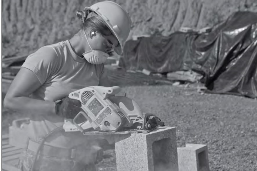
A Soldier uses a circular saw to cut a block for a bond beam.
