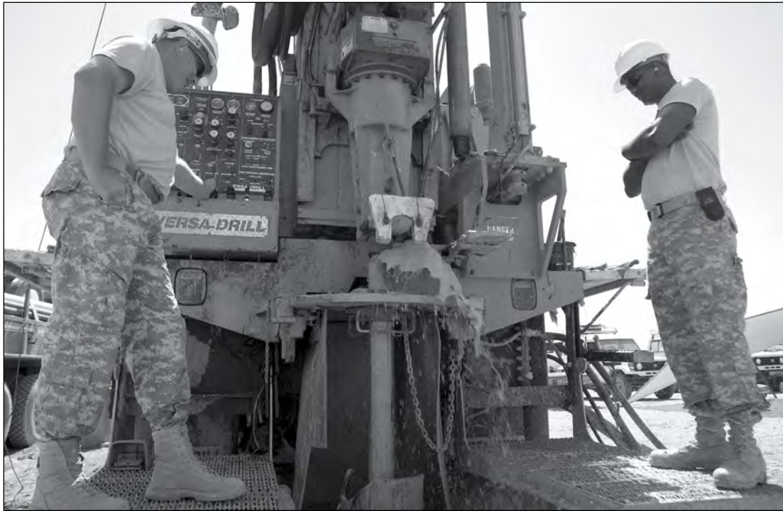
Soldiers from the 775th Engineer Detachment (Well Drilling), drill a well in Djibouti in support of Combined Joint Task Force–Horn of Africa.
