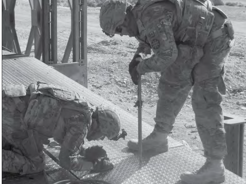
Soldiers from the 1438th MRBC inspect decking on an overbridge ramp.
