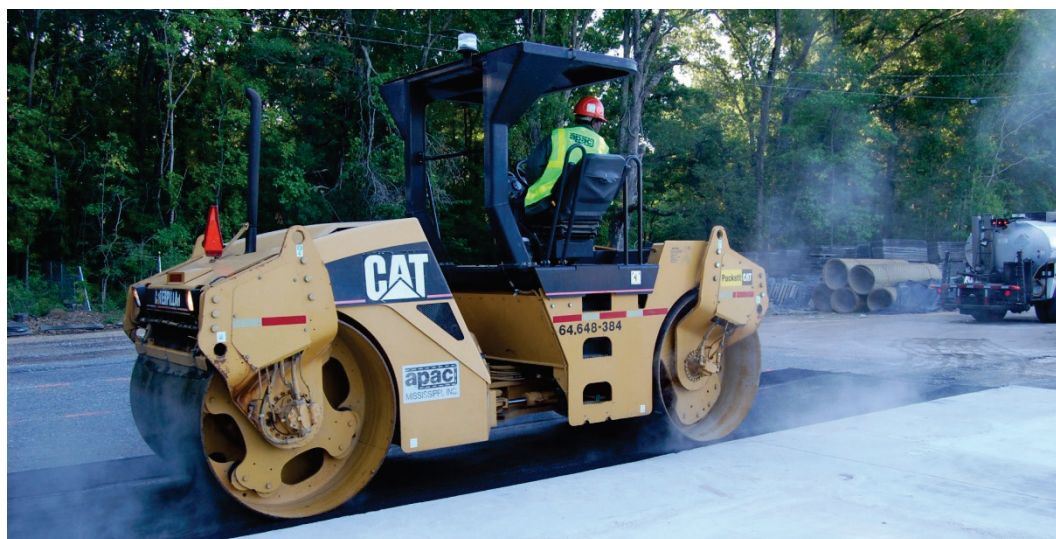
Figure 6. HMA compaction with a double drum vibratory compactor.
