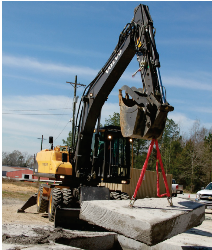
Figure 34. Removing with the excavator.
