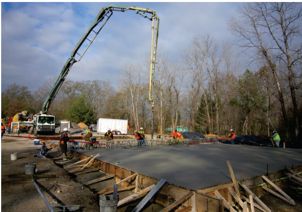
Figure 5. PCC placement.
