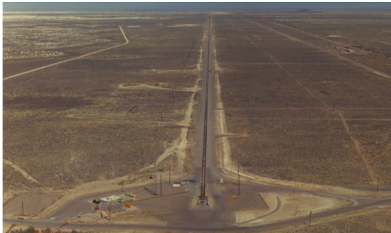
Figure 2: Holloman High Speed Test Track, Aerial View.
