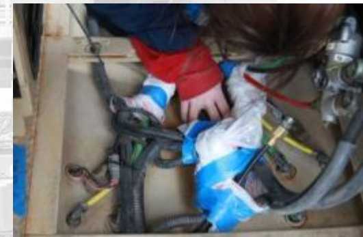
Hand sanding to roughen existing, intact coating
