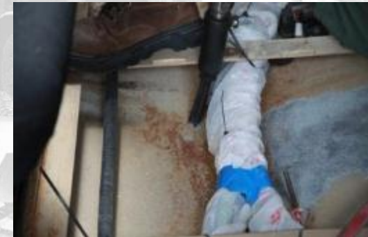
Needle gun cleaning of corrosion and loosely adherent coating
