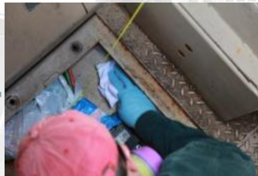
Final solvent wipe after vacuuming to remove all remaining debris
