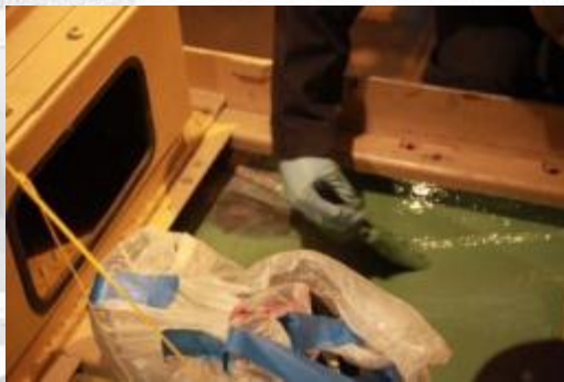
Brush application of coating, 2 coats, recommend using contrasting colors
