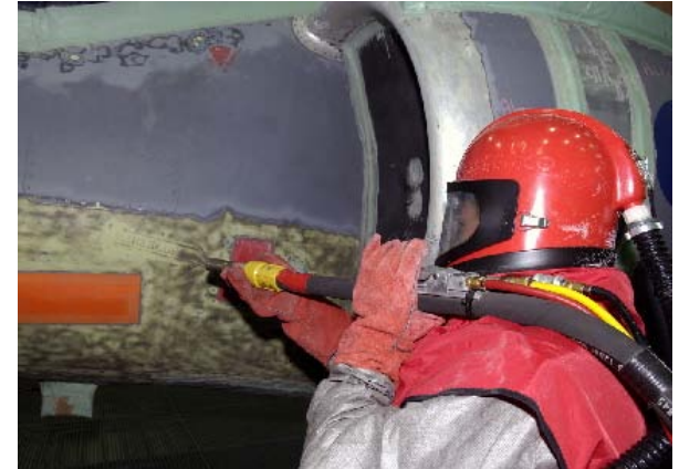
Plastic Media Blasting
