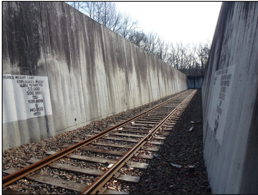
Figure 42. View of interior of barricaded Railroad Siding, Group A and B barricades
