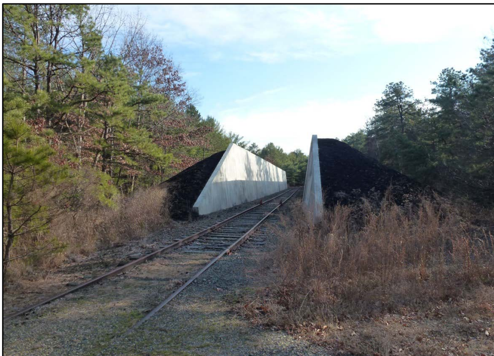
Figure 9. Barricaded railroad sidings still utilized but not as originally designed; no longer able to enter both sides of the siding
