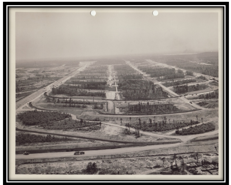
1944 aerial Army Area barricades
