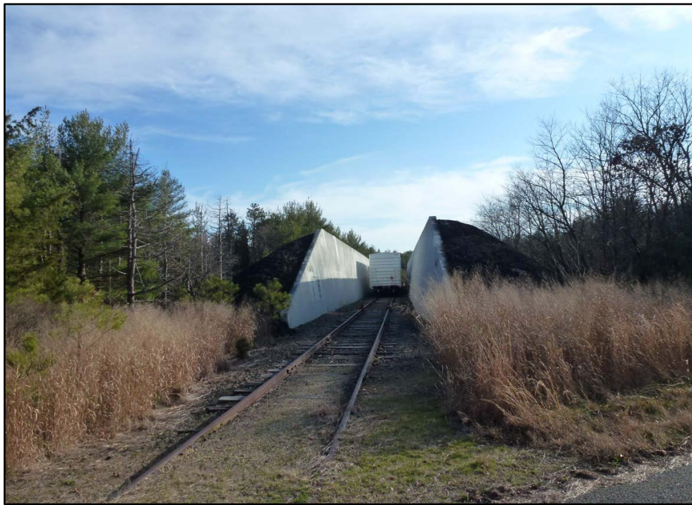
Figure 8. Refurbished barricaded railroad siding
