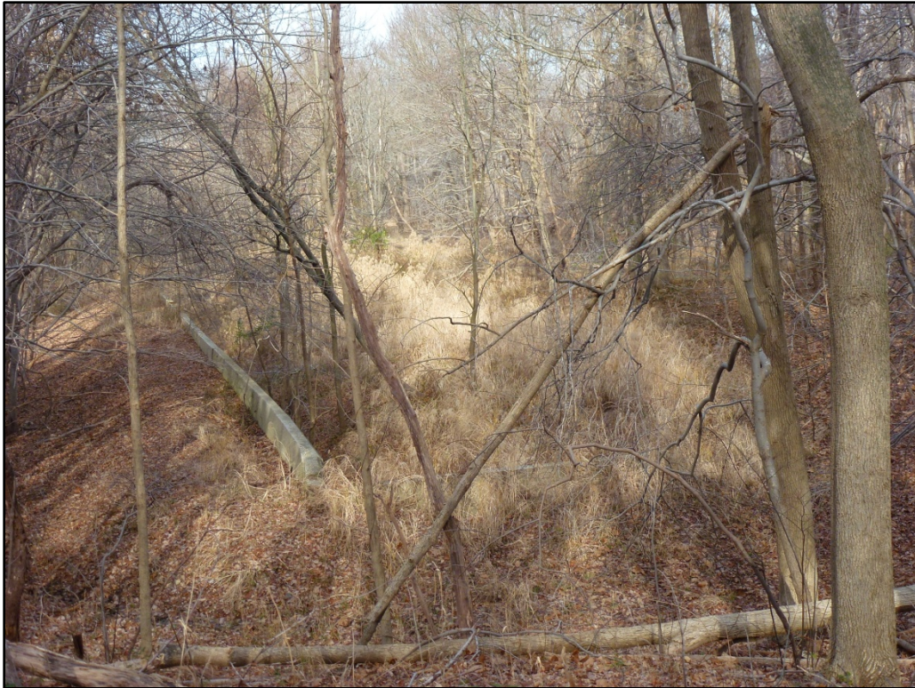
Figure 27. View of barricaded railroad siding
