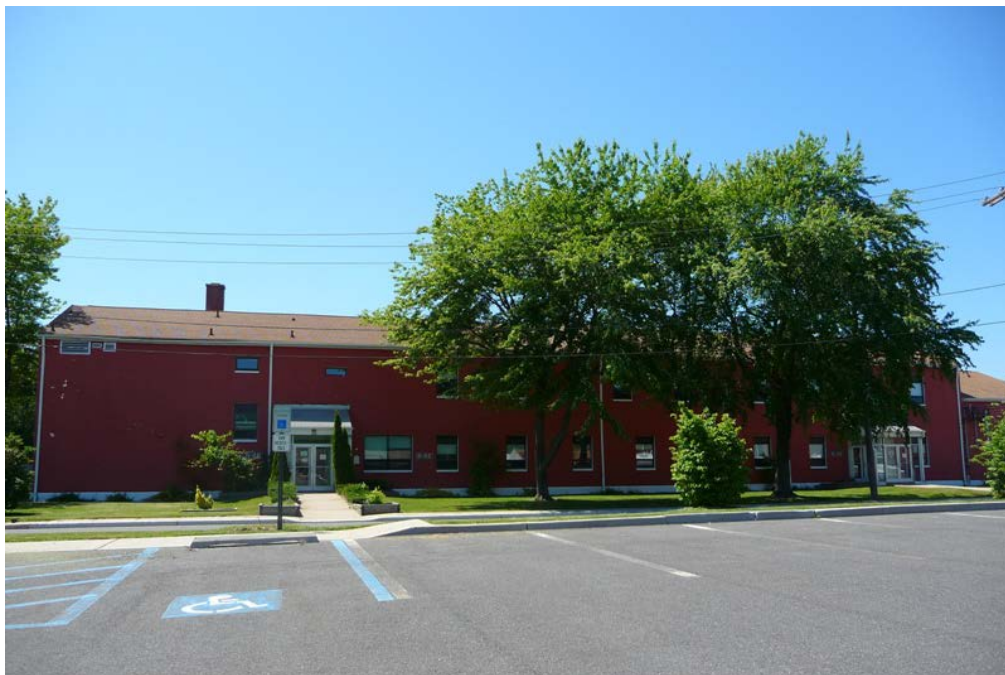
Figure 31. Example of integrity changes to buildings in the Waterfront Administration Area with removal of fenestration and addition of new entrances and doors (ERDC-CERL, 2010).
