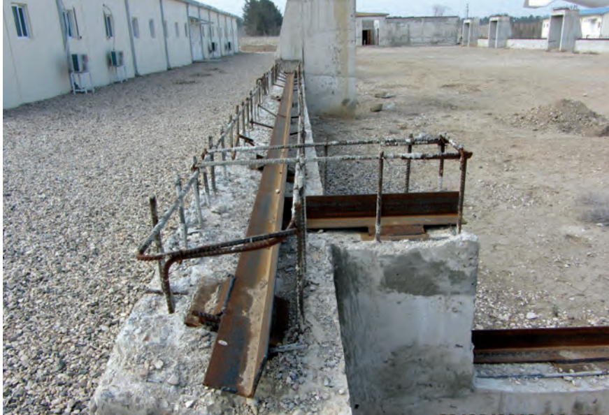
A SIGAR inspection of Camp Monitor found that the dining-facility construction was limited to the concrete footings that appeared to be of poor quality, with uneven and cracked concrete surfaces. (SIGAR photo)
