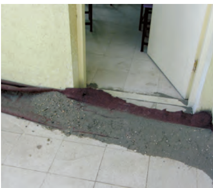
SIGAR auditors discovered a second floor terrace that slopes toward the classroom door, requiring an improvised dam to stop rainwater from flowing into the classroom. (SIGAR photo by Les Thompson)
