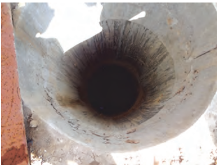
Neither access point to the septic tank has a solid cast iron cover or a permanent ladder, both of which are required by the contract. (SIGAR photo by Ron Riach)
