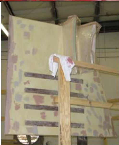
Installation of Vertical Shear Ties
