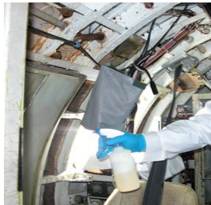
Cleaning Mildew Growth by Spraying Mildew Remover
