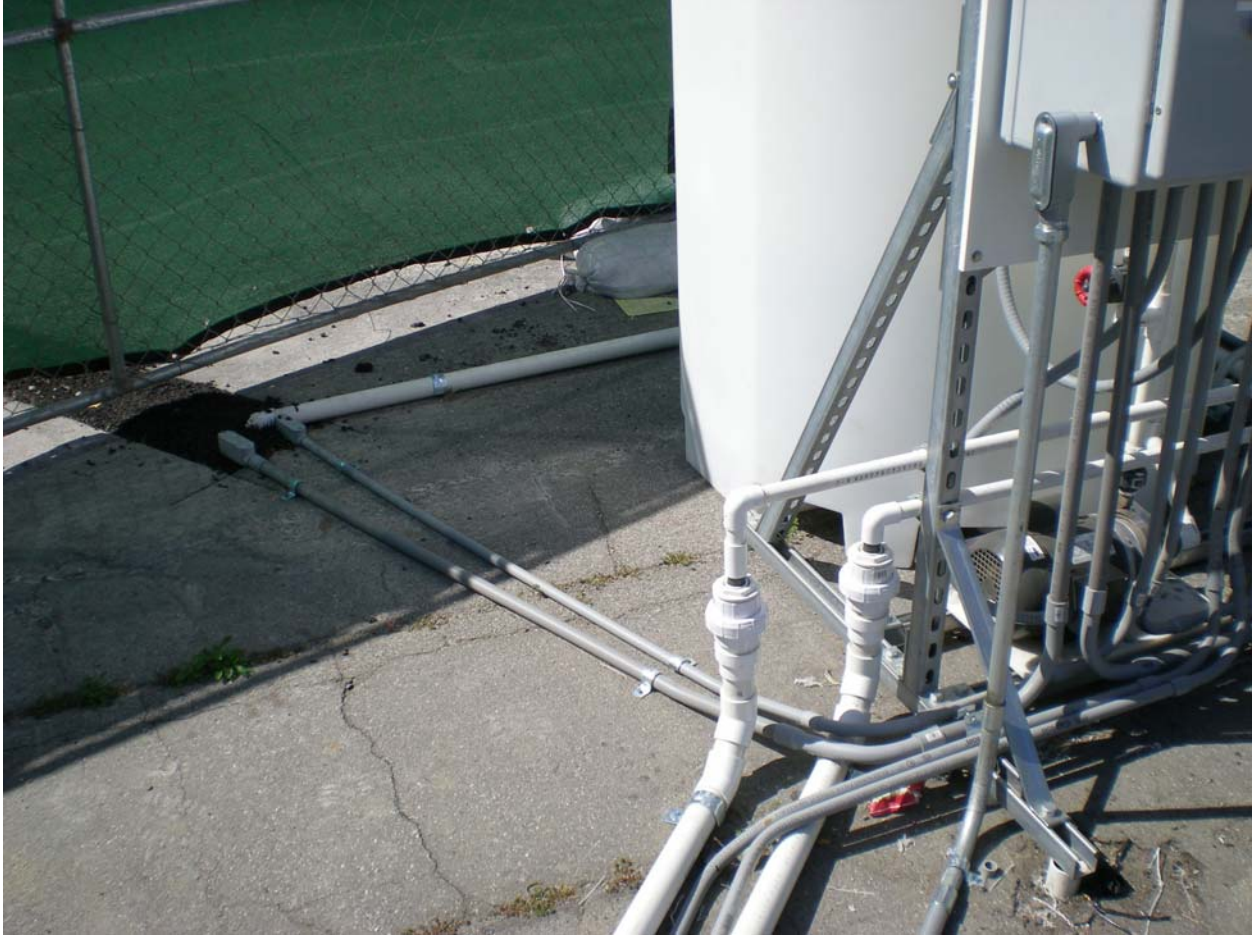
Picture 5. Extraction piping daylighting.
