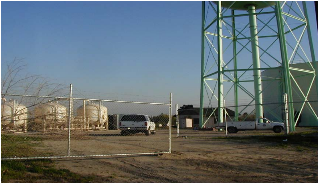
Figure 10. City of Colton, Dominick Reservoir, and Wells #15 and #17 treatment system.
