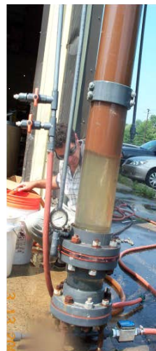
Resin being removed through unscreened mid-lateral.
