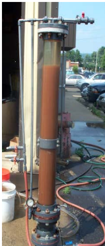
6" Pilot column before flow applied
