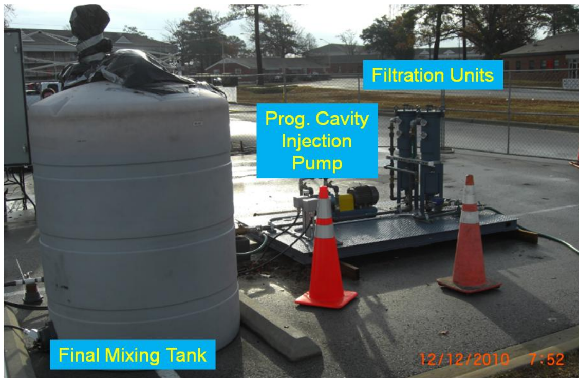
Figure 5-15. Fluid injection and filtering system.
