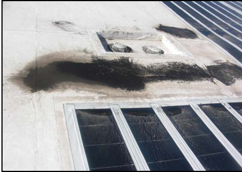
Figure-47: Severe, localized mold growth due to water ponding before it reaches the drains.
