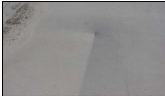
Figure-28: Mold growth (upper left corner) and warping dens-deck (center) at Site II (NAS Patuxent River).
