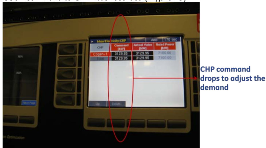
Figure 23: U90+ commands CHP during islanding
