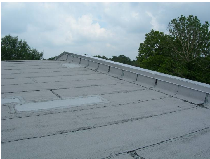
Figure A-3, 5 Old Sloped Built Up Roof on Gym
