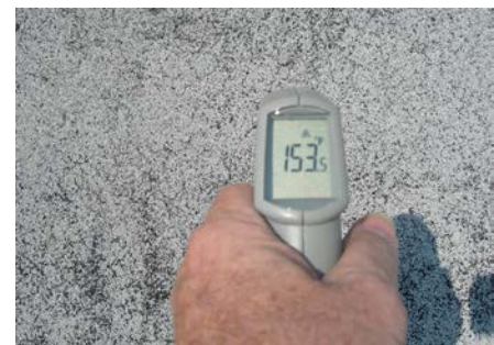
Figure A-3, 15 IR Surface Spot Temperature
