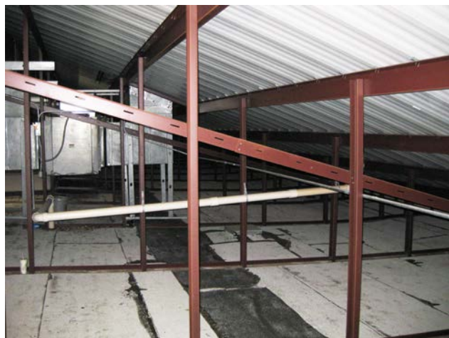
Figure A-6, 2 Slope Build Up Metal Re-roof Over BUR
