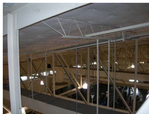
Figure A-3, 4 Gym Interior Ceiling
