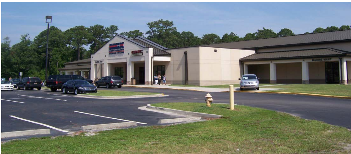
Figure 4.1-2 Building 1283, Base Exchange at MCAS Beaufort.
