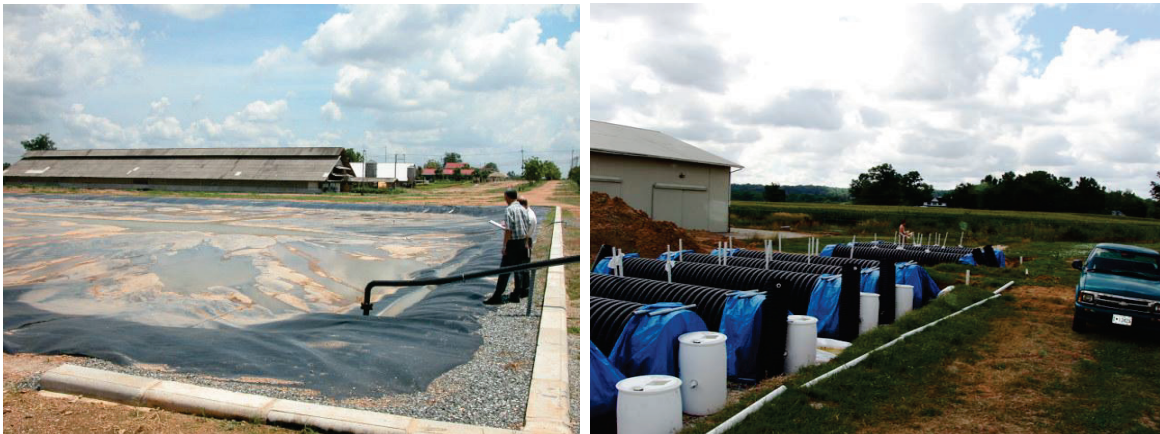
Figure 4. Two examples of simple anaerobic digester reactors: covered lagoon (left) and bag reactors (right) (from Lansing and Moss 2010).
