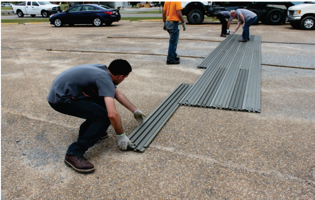
Figure 13. MLC-70 panel assembly.
