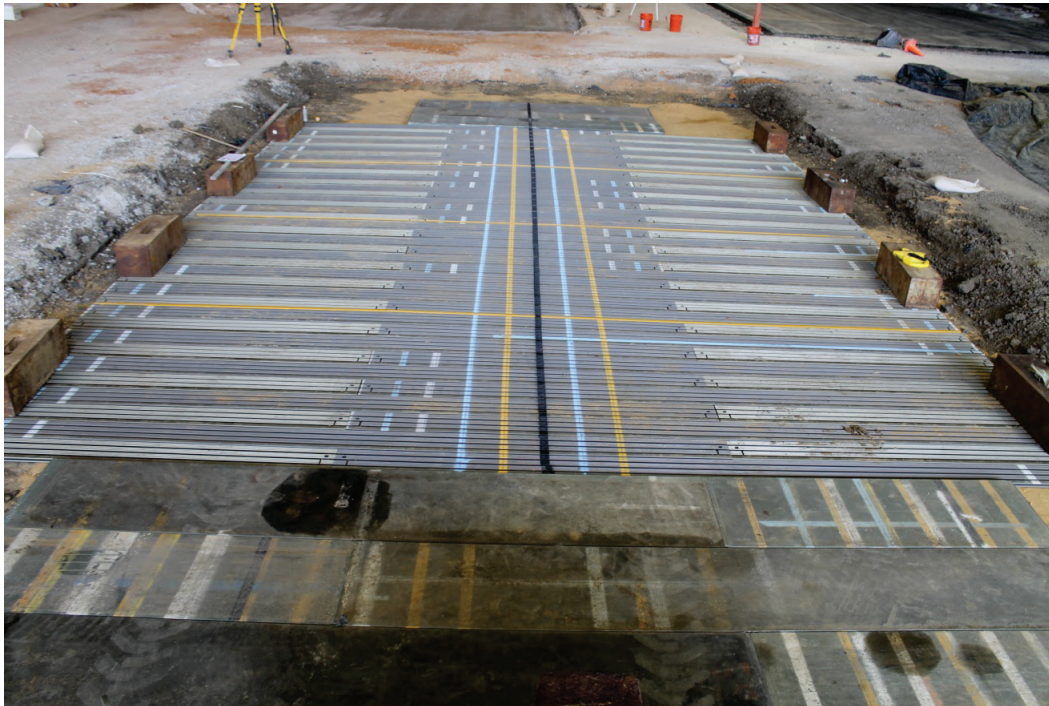
Figure 20. Final assembled 25 CBR test section.
