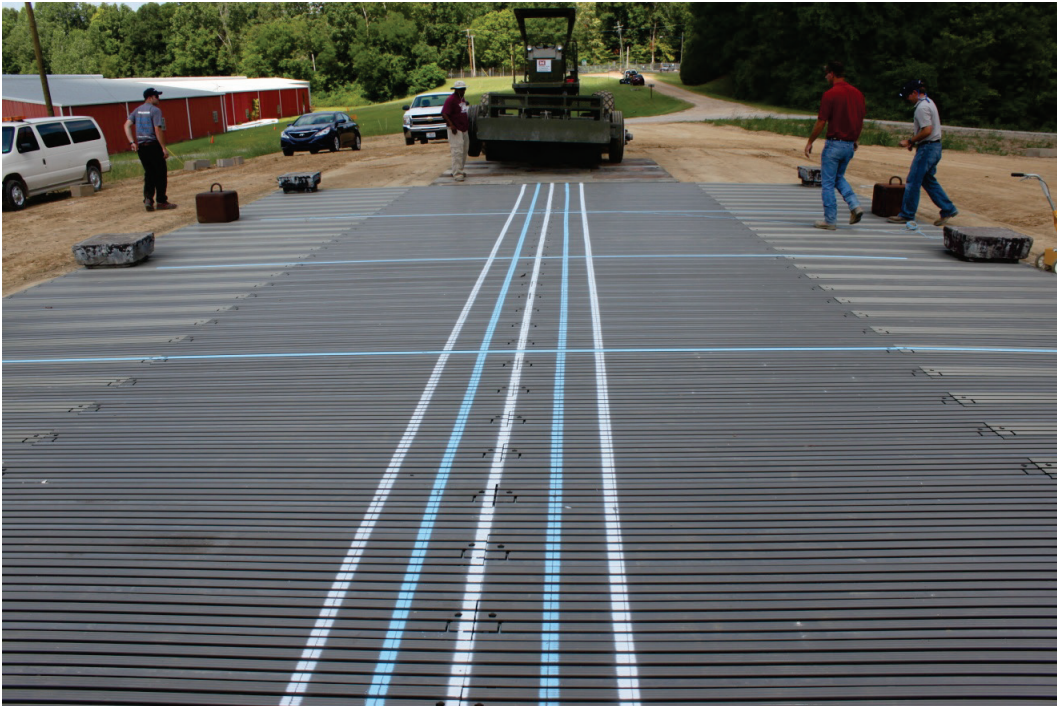
Figure 19. Final assembled F-15E traffic area with AM2 ramps.
