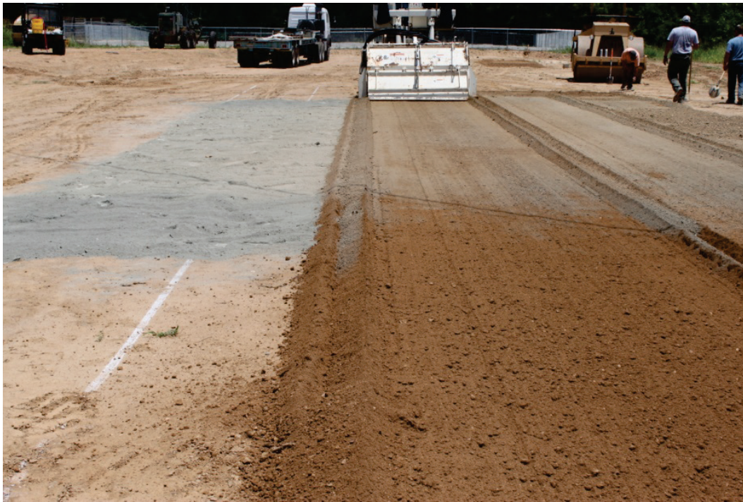
Figure 10. Mixing cement into the soil with a reclaimer/mixer.
