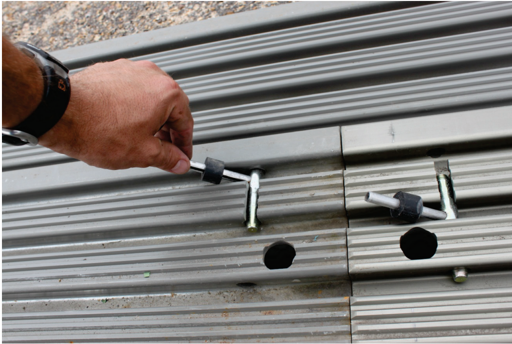
Figure 14. MLC-70 shoot bolt insertion.
