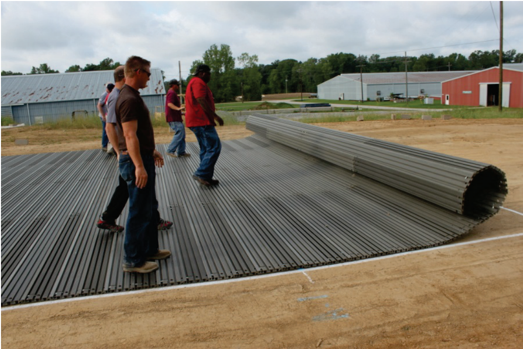
Figure 18. Unrolling MLC-70 matting on prepared test section.
