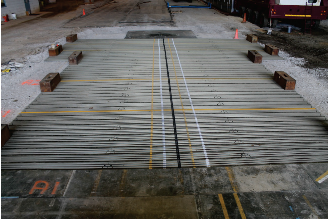
Figure 21. Final assembled 100 CBR section.
