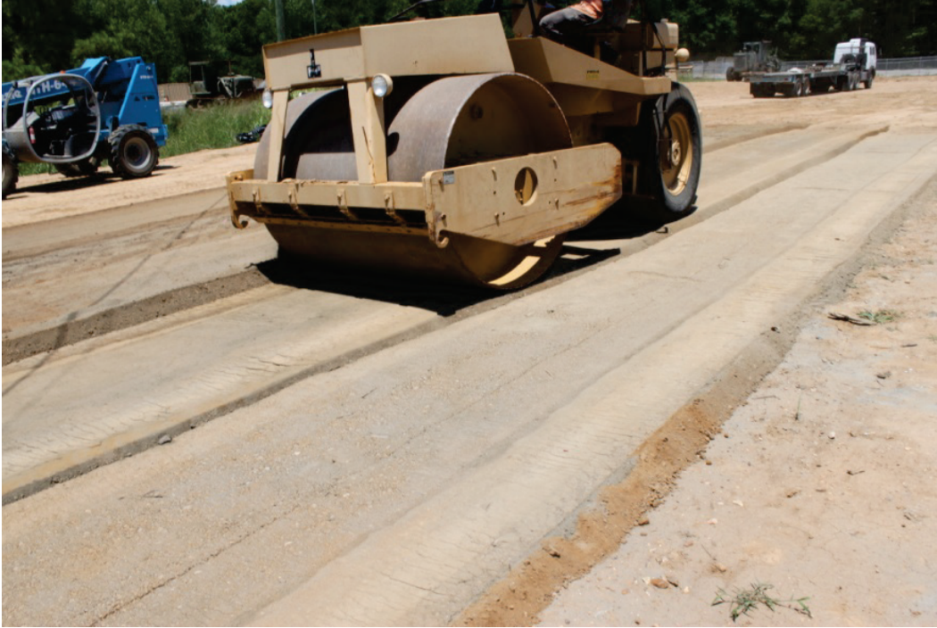
Figure 11. Compacting stabilized subgrade with vibratory steel wheel roller.
