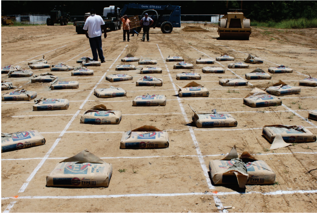
Figure 9. Cement bags placed in grid area prior to spreading.
