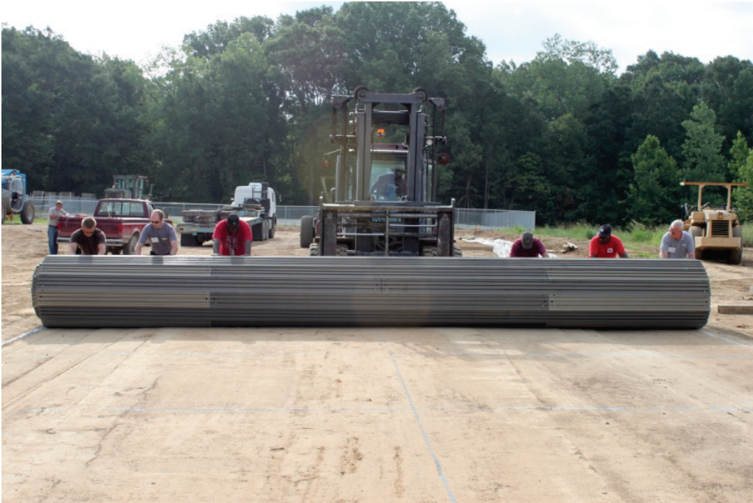
Figure 17. Unrolling MLC-70 matting on prepared test section.
