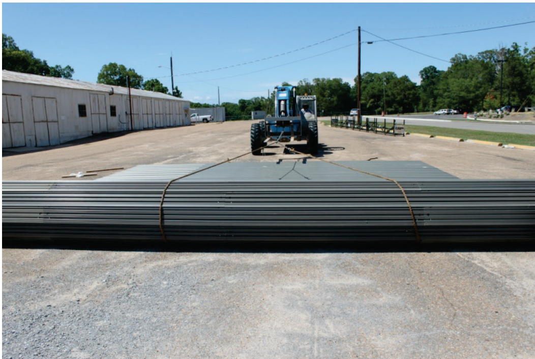
Figure 15. Rolling assembled mat expense for transportation to the test section.
