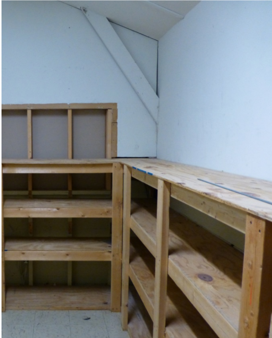
Figure 19. An example of an exposed structure (ERDC-CERL, 2013).
