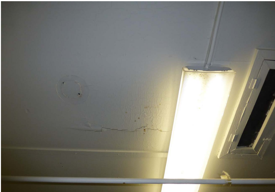
Figure 44. Example of an electrical box (center, left) marking the location of an original light fixture (ERDC-CERL, 2013).
