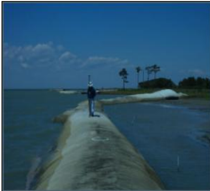
Figure 3. Geotextile tubes fully inflated, before placing dredged material, western side of Barren Island (photo 2000).
