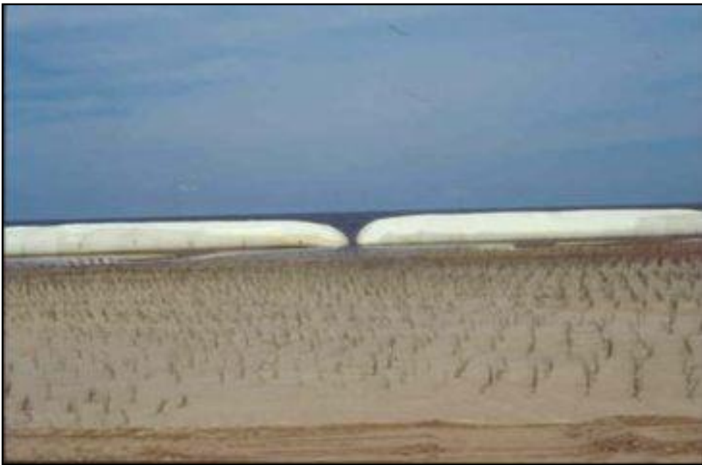
Figure 5. Wetland species planted on dredged material behind geotextile structure, western side of Barren Island (photo 2000).
