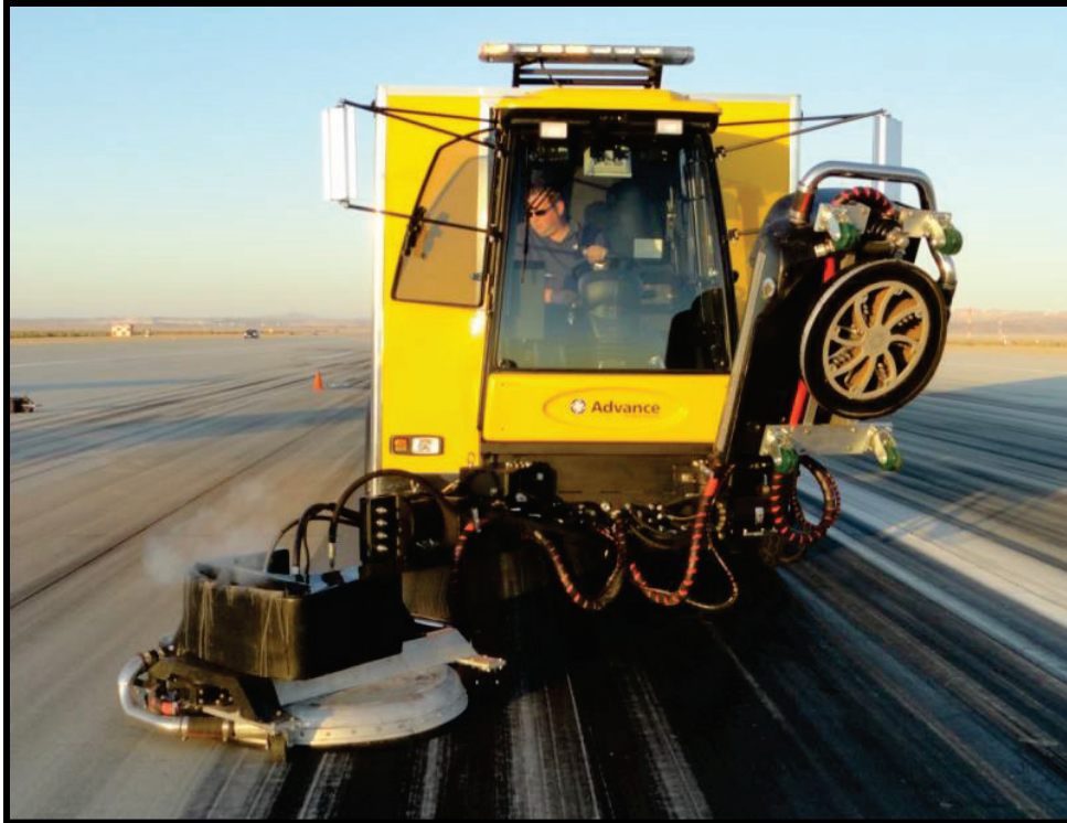
Figure 68. Cyclone 4006 removing rubber on Runway 22L.
