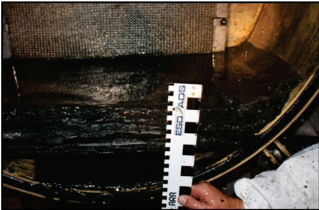
Figure 73. Solids collected in a Trackjet vacuum chamber.
