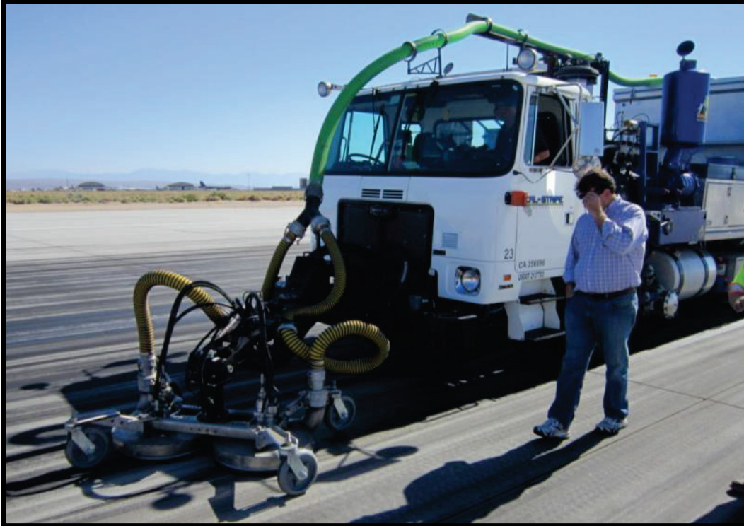
Figure 74. SH8000R removing rubber on Runway 22L.
