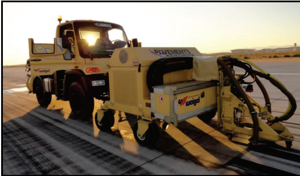
Figure 71. Trackjet removing rubber on Runway 22L.
