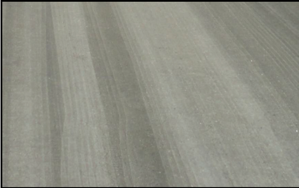
Figure 24. Typical pavement surface on Runway 22L after Cyclone 4006 rubber removal.
