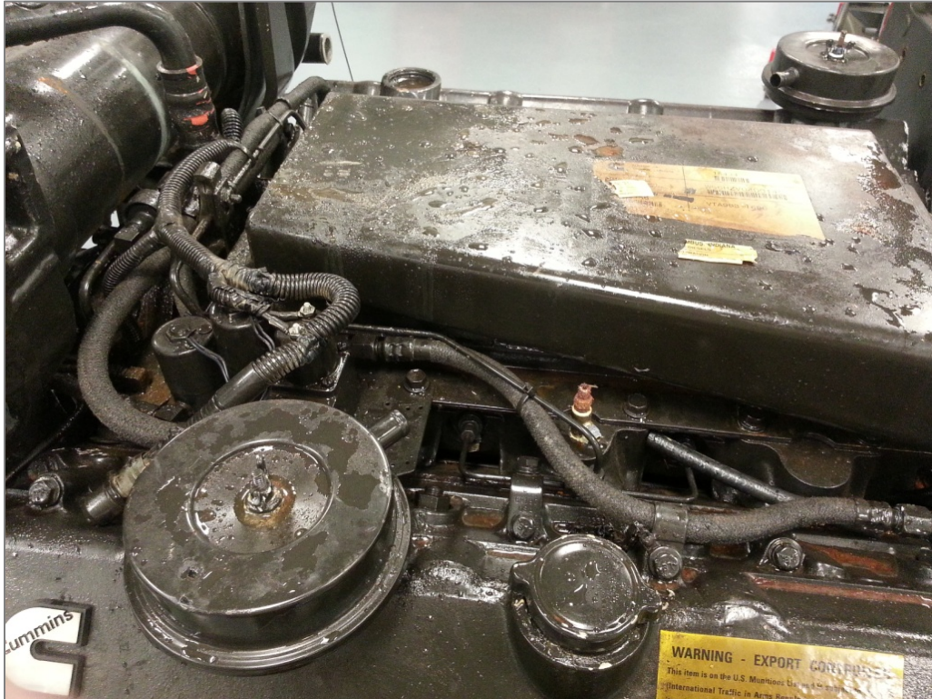
Figure 3. Moisture Accumulated on Engine in Container
