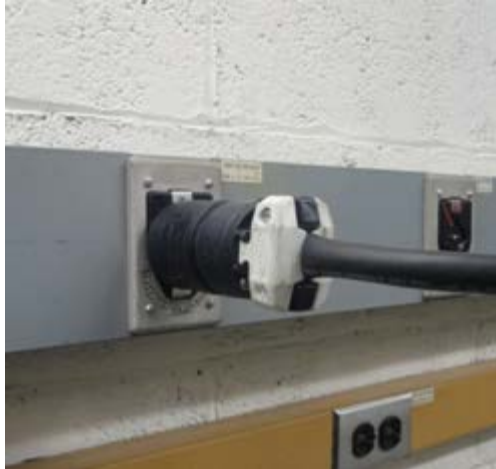
Figure C-14 240 V AC Outlet for EMA
