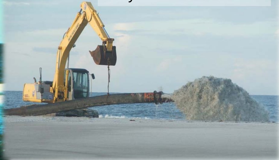
Hydraulic Placement
