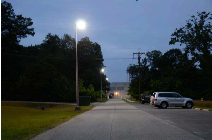
Figure 16. Light quality of the LED streetlight, taken on June 11, 2012 at 8:53pm (100% intensity).
