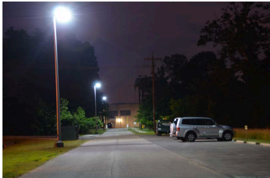
Figure 17. Light quality of the LED streetlight, taken on June 11, 2012 at 9:14pm (80% intensity).
